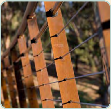
Balustrade in stainless steel and weathering steel
