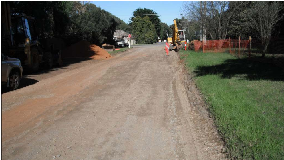
Photo of drainage works being installed
