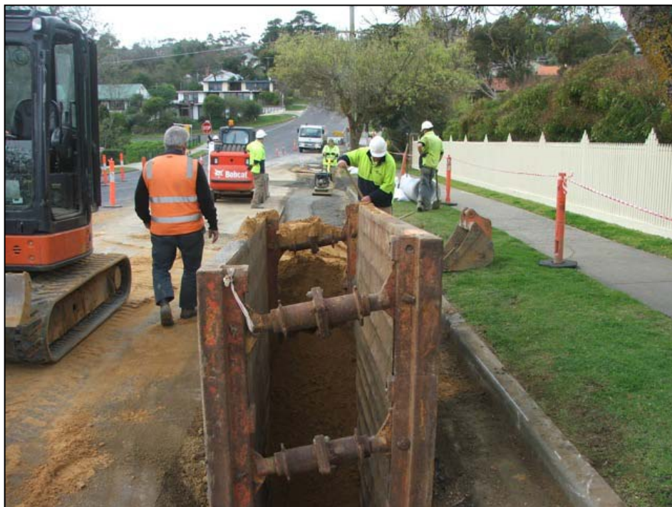
Photo of new drainage line being installed within Barkly Street
