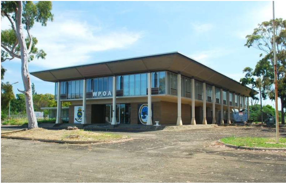
Figure 7: Former BP Refinery/Administration Building
