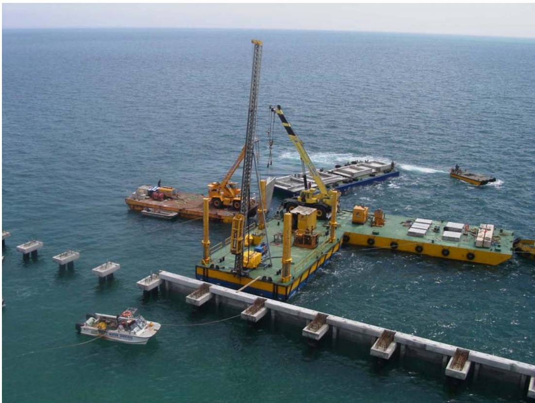
■ Figure 2-13 Likely Construction Activities During Wavescreen Construction
