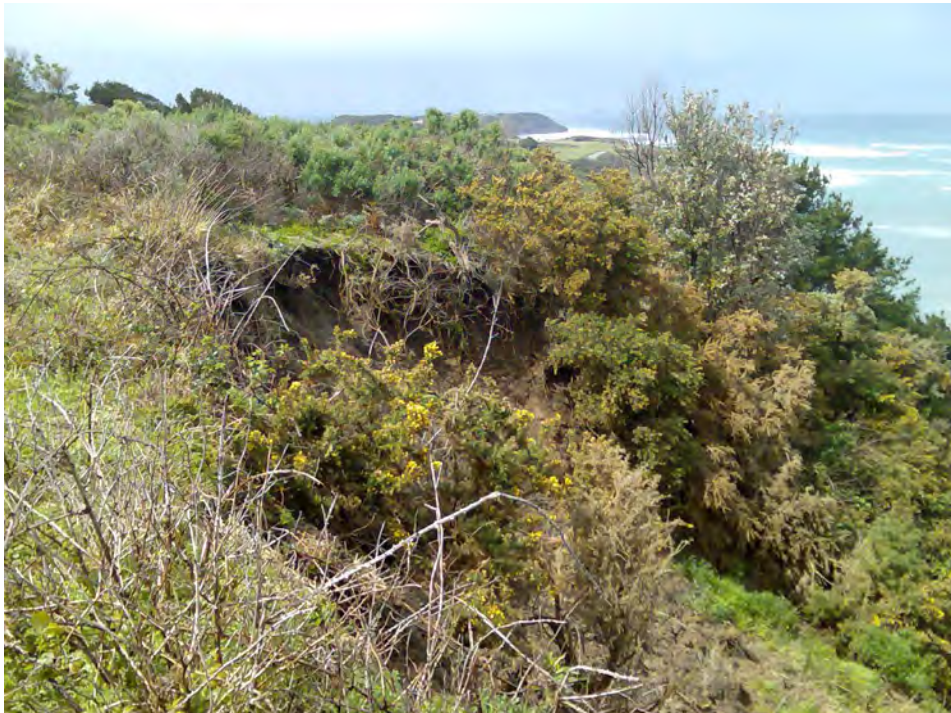
Plate 12.2: Scarp with Active Erosion and Movement
