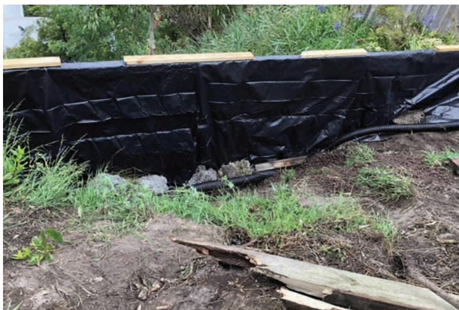
FIGURE 3.8: CONSTRUCTION OF ORIGINAL RETAINING WALL INSTALLED BY THE BORGHESI. 96
