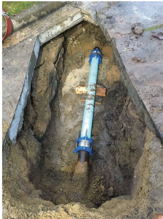
FIGURE 3.15: PHOTO OF THE PIPE POST REPLACEMENT. 126
