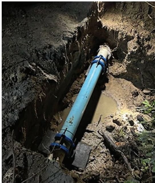
FIGURE 3.32: PHOTOGRAPH OF REPAIRED SECTION OF THE BURST WATER MAIN. 476
