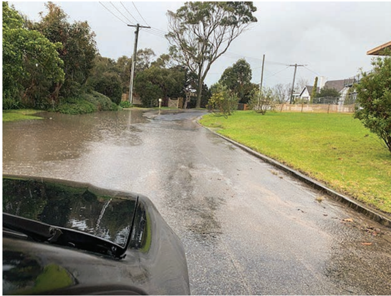
FIGURE 3.10: FLOODING IN FRONT OF 11 PROSPECT HILL ROAD. 103
