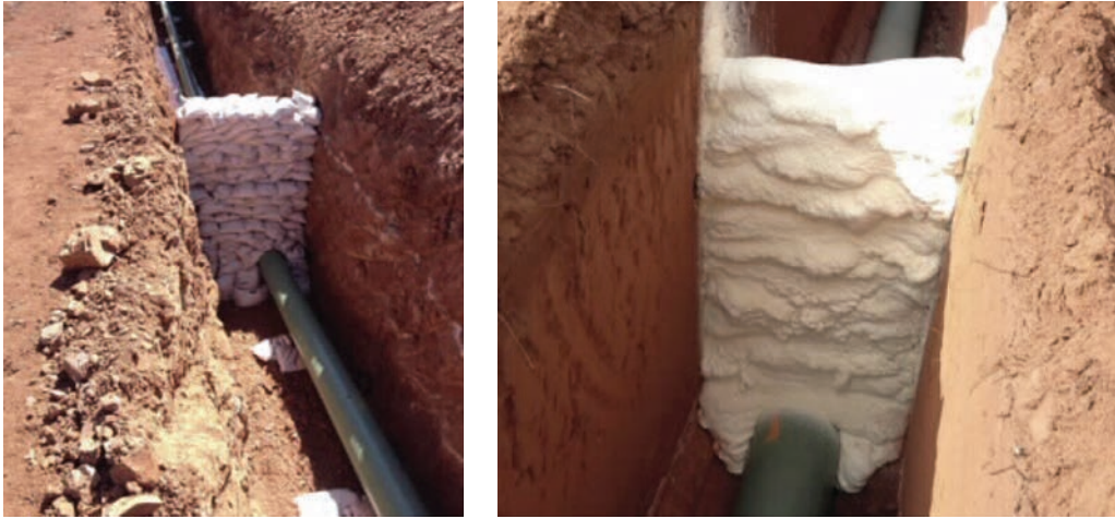
FIGURE 5.9: EXAMPLES OF TRENCH STOPS. 110
