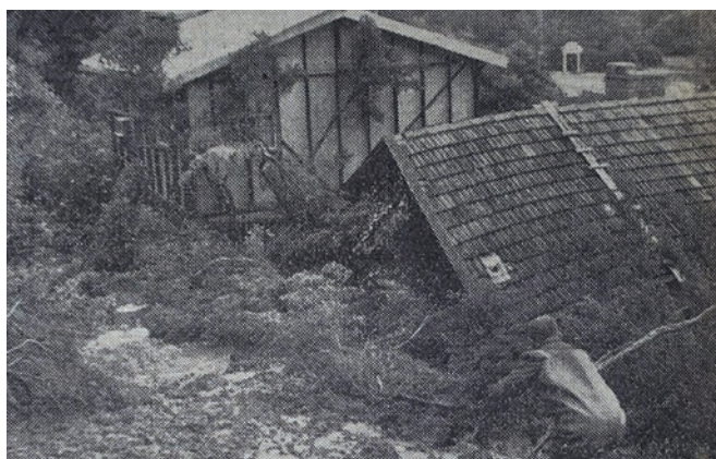
FIGURE 3.1: VIEW LOOKING WEST AT 565 POINT NEPEAN ROAD SHOWING DAMAGE TO DWELLINGS FROM LANDSLIDE DEBRIS. 5
