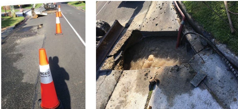
FIGURE 3.13: IMAGES OF THE CUT TO THE ROAD SURFACE AT COBURN AVENUE. 124
