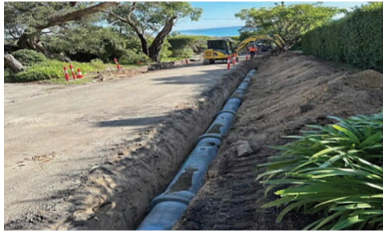
FIGURE 3.24: SHIRE'S STORM WATER UPGRADE ON VIEW POINT ROAD. 299
