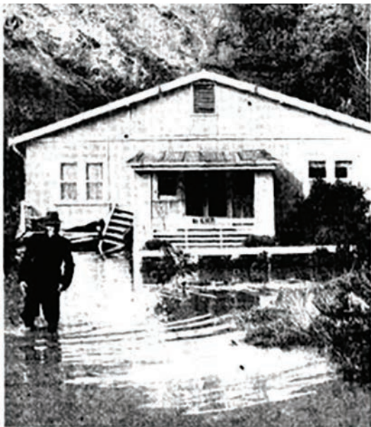
THIS HOUSE, The Rocks, at the foot of Arthur's Seat was pushed forward 10 feet by a landslide today. It collapsed on its basement garage, smashing it to matchwood. See story page one.
