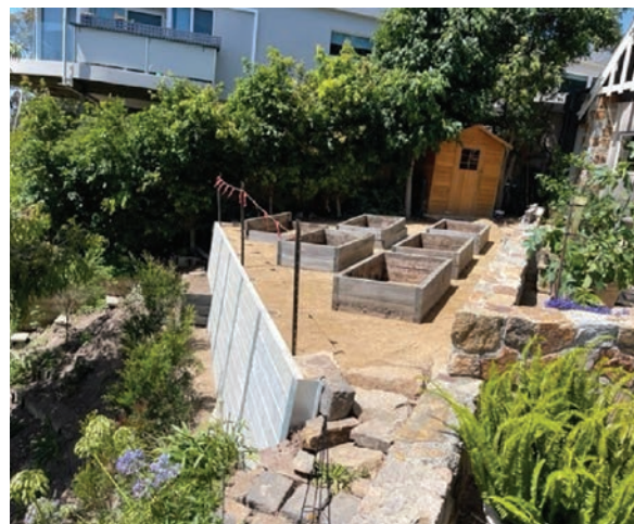
FIGURE 3.27: COMPLETED REINFORCEMENT WALL AT 10–12 VIEW POINT ROAD. 341
