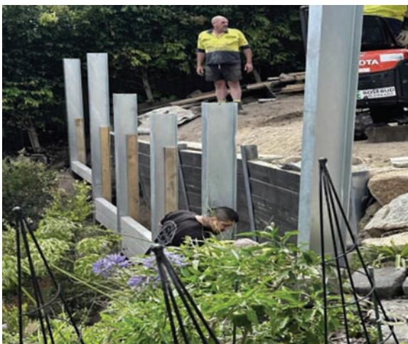
FIGURE 3.26: CONSTRUCTION OF THE REINFORCEMENT WALL AT 10–12 VIEW POINT ROAD. 340
