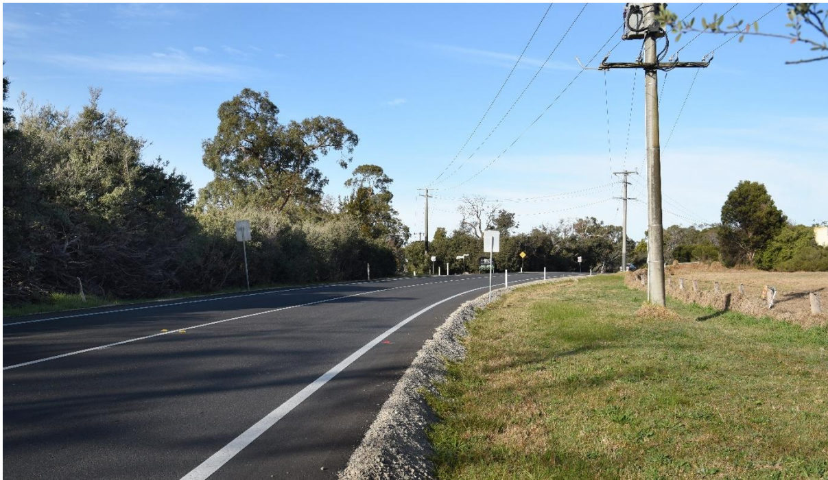
Figure 11-2 Existing view from Tyabb-Tooradin Road
