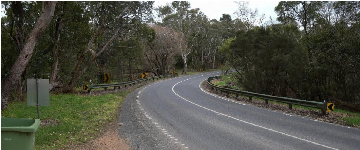
Figure 9-3 Existing view from Main Creek Road
