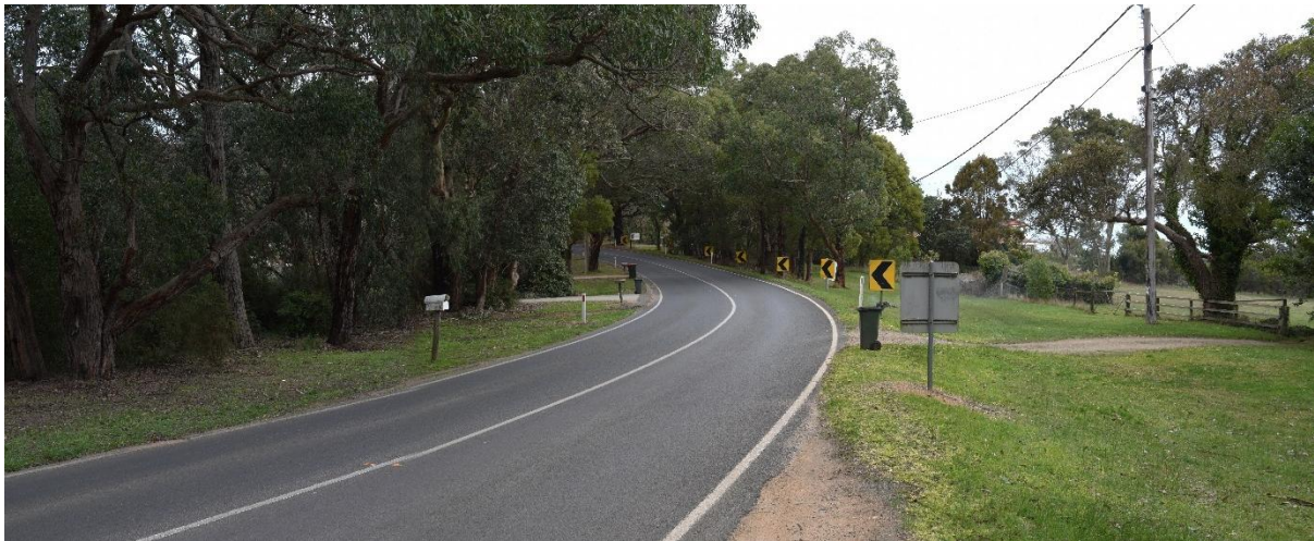
Figure 9-7 Existing view from Main Creek Road
