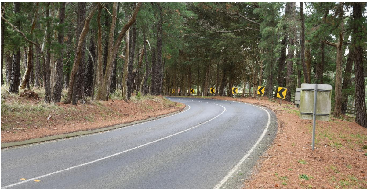
Figure 9-5 Existing view from Main Creek Road
