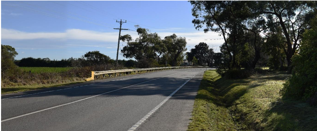
Figure 11-4 Existing view from Tyabb-Tooradin Road
