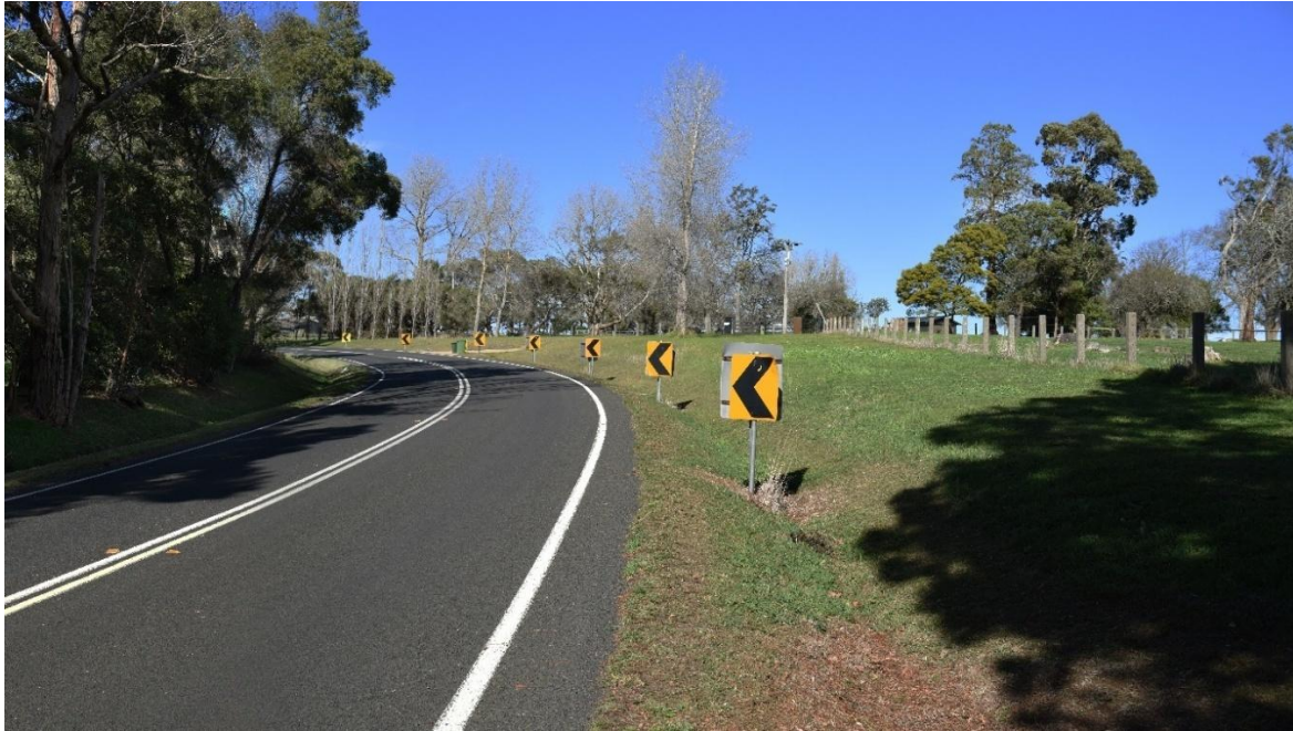
Figure 6-2 Existing view from Baldrys Road
