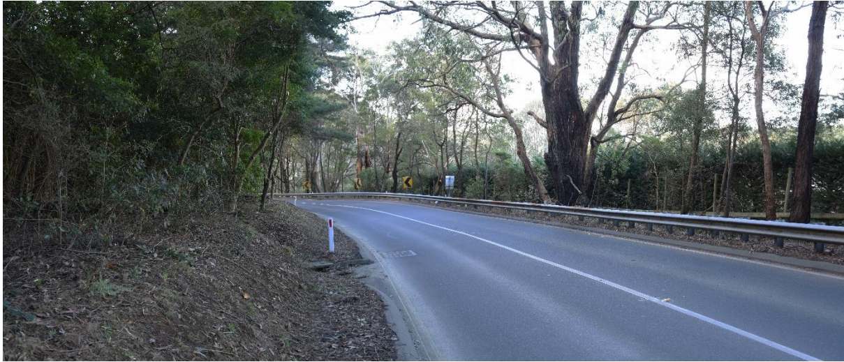
Figure 10-4 Existing view from Shands Road
