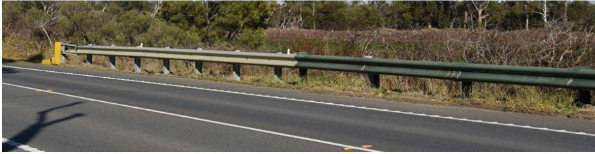
Figure 13-5 Road safety barrier along Tyabb-Tooradin Road
