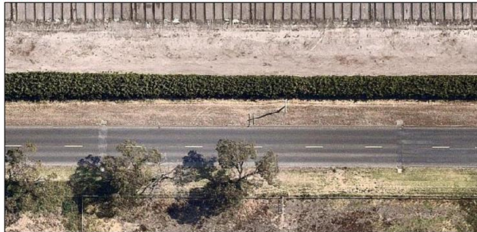
Figure 3.3 Bungower Road – Typical Existing Configuration
