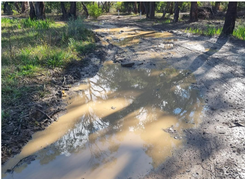
Figure 11 – Water pooling at the Glossop Street / Creswell Street intersection (facing west).
