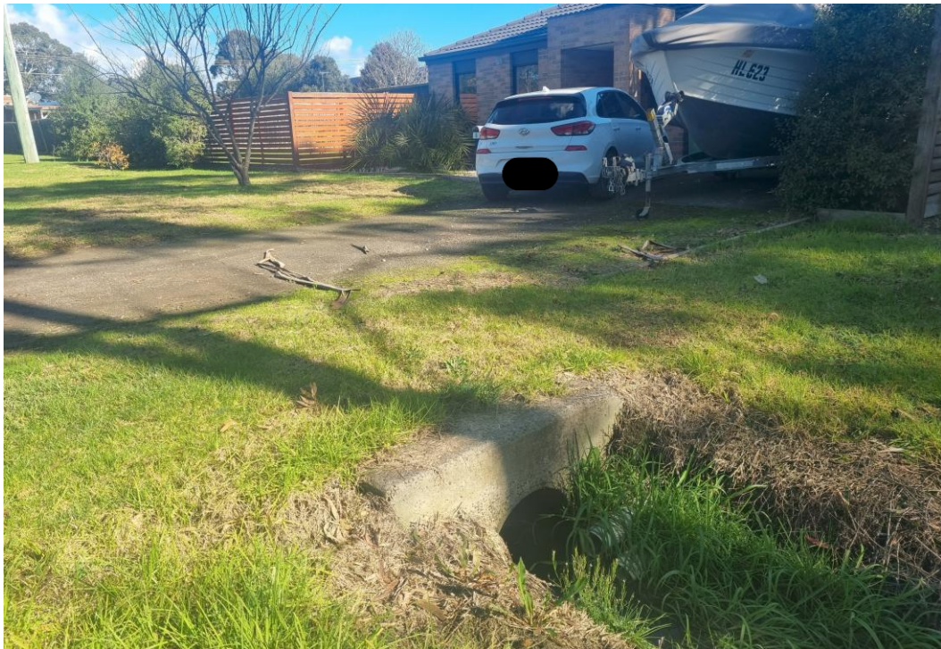
Figure 06 – Conversion from drainage pipes to open channel drainage adjacent to 6 Cooma Street.
