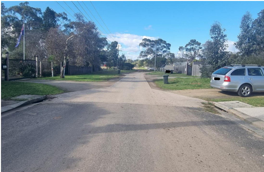
Figure 14 – The existing transition from formalised road reserve to single carriageway within Creswell Street.
