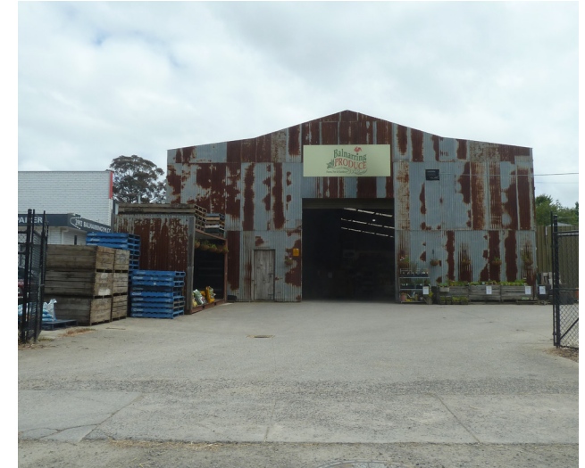
06 Balnarring Industrial Shed
