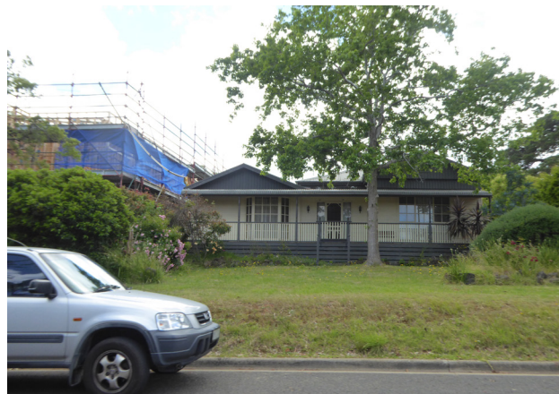
212 Mount Eliza - construction of larger new development
