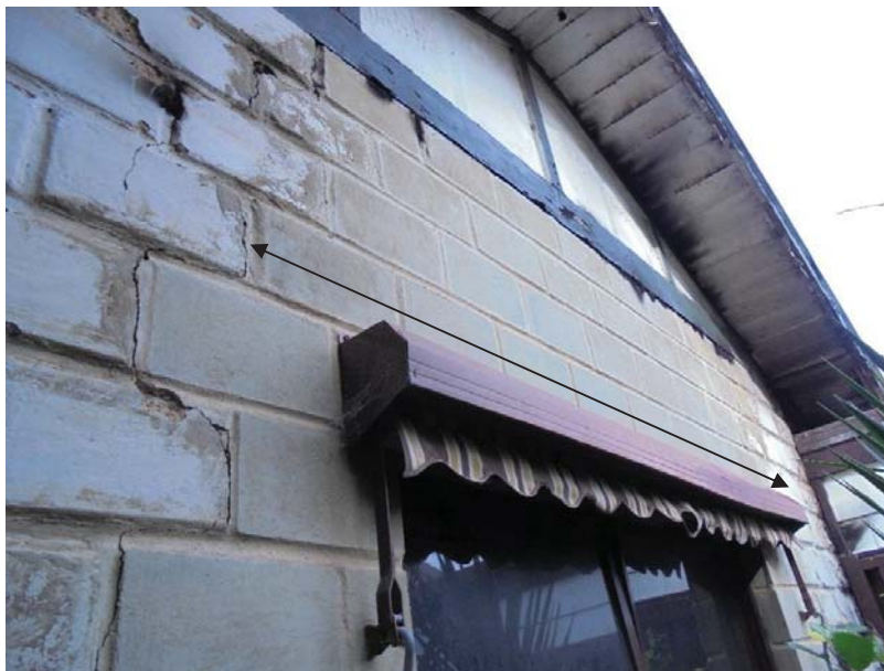
Previous repairs to walls
