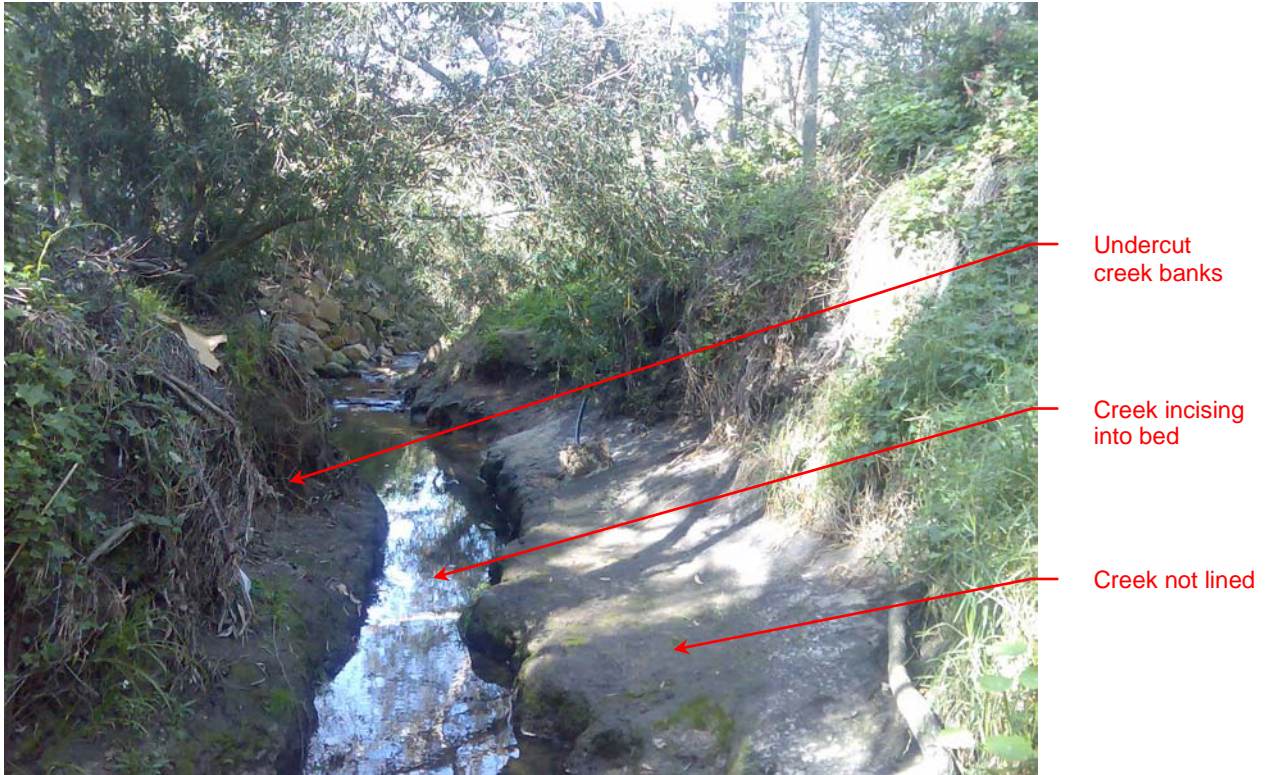
Figure 9-7: Undercut banks to rear of 9-11 Marchington Avenue
