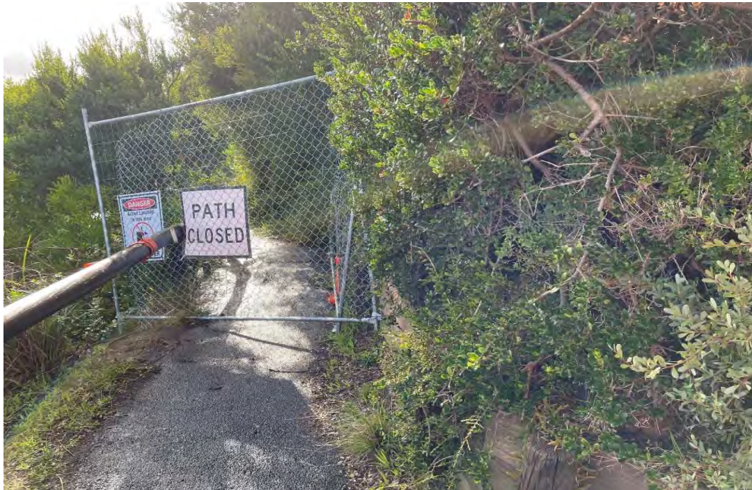
Figure 6-2 – Fencing on the southern side of the active failure in Section 7
