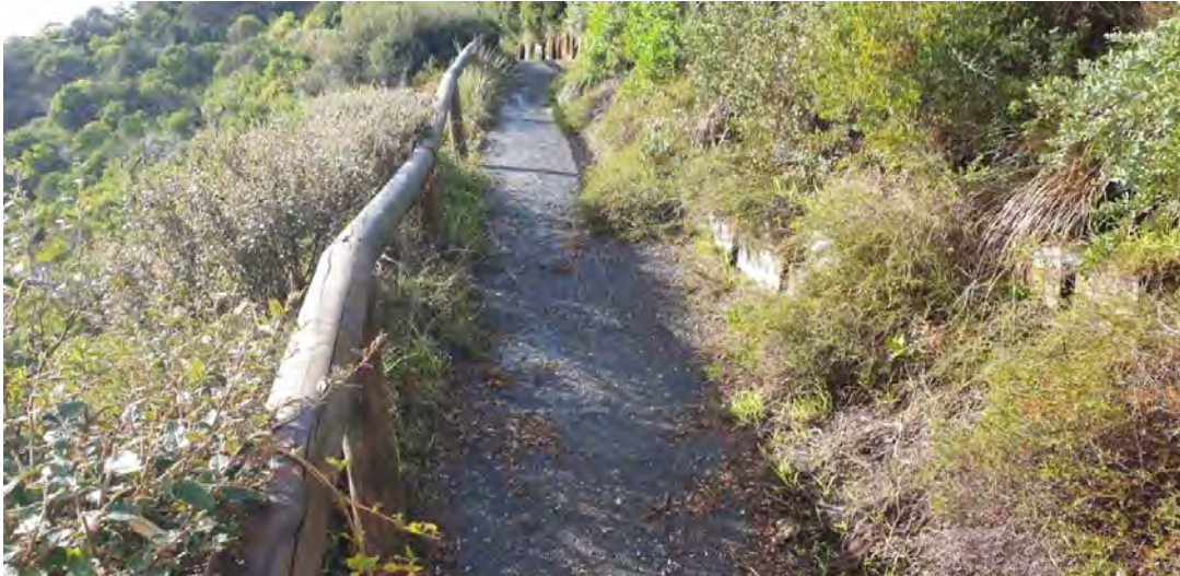
Figure 4-4 – Example of path built on fill embankment (Section 9)
