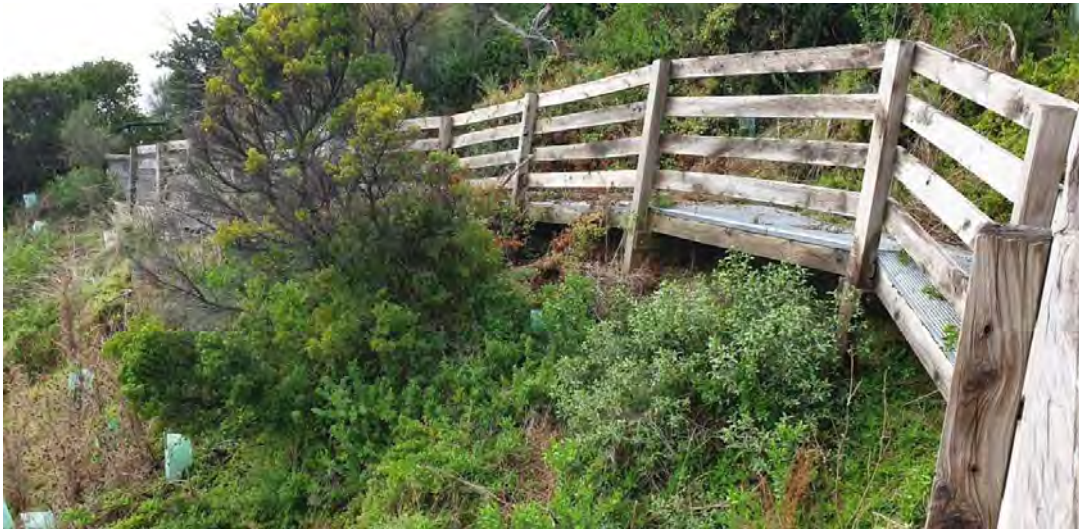
Figure 4-13 – The Hump Bridge (Section 18)
