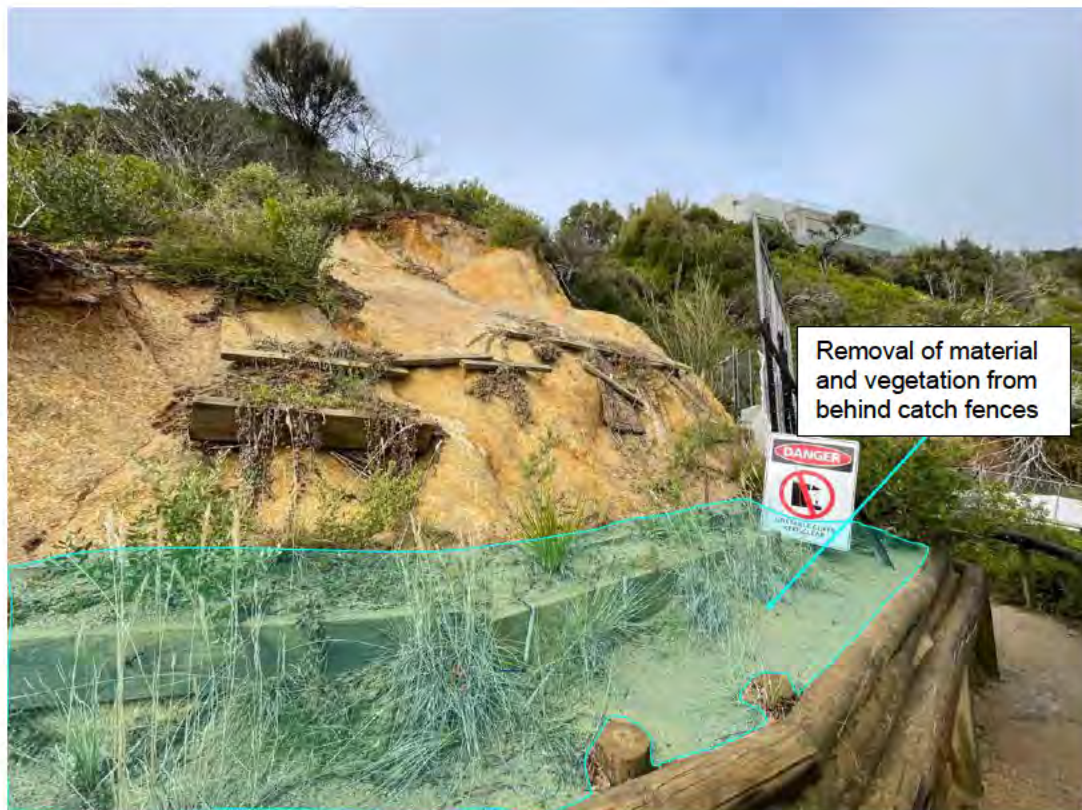
Figure 6-7 – Section 19: material and vegetation to be removed from behind catch wall
