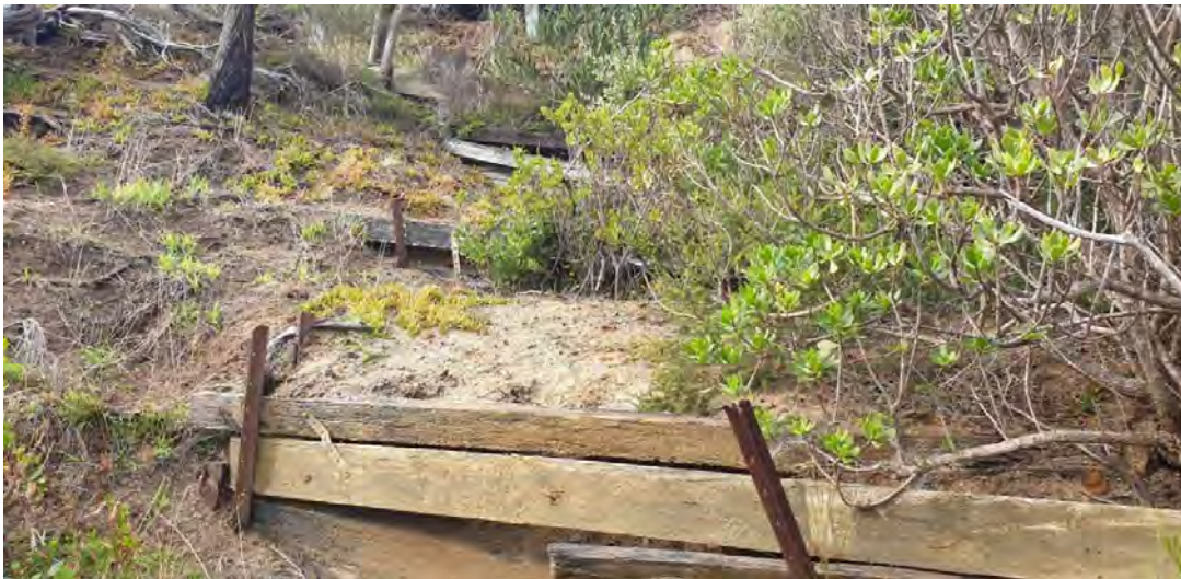
Figure 4-9 – Example of informal retaining walls (Section 11)
