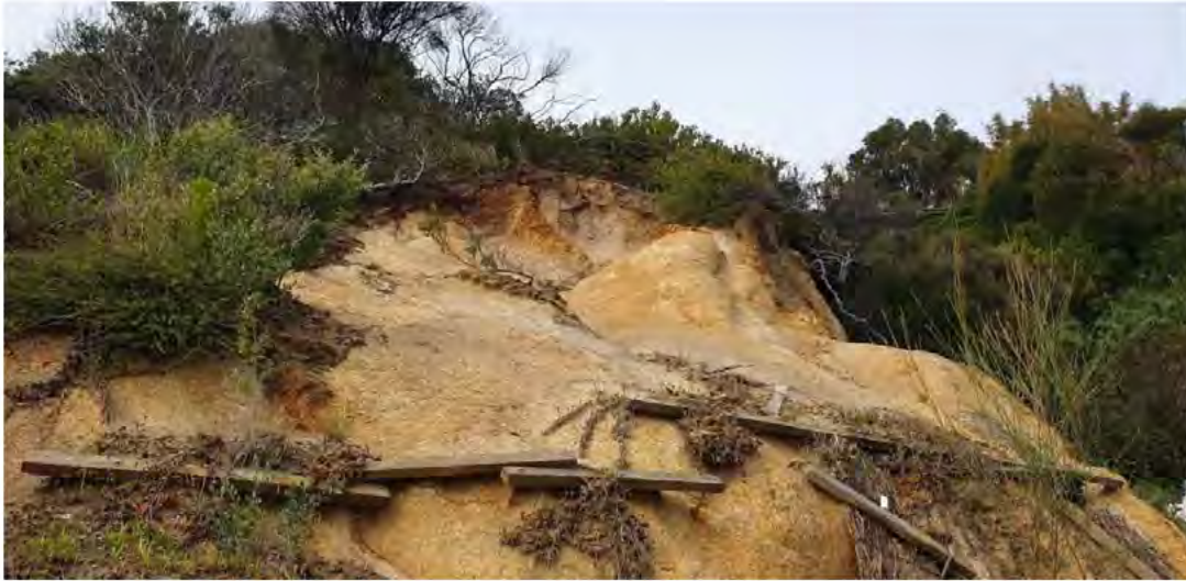
Figure 4-15 – Informal remedial works in Section 19
