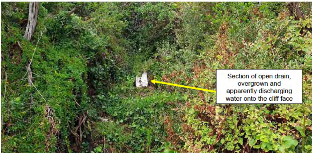
Figure 4-16 – Section of open drain (Section 18).
