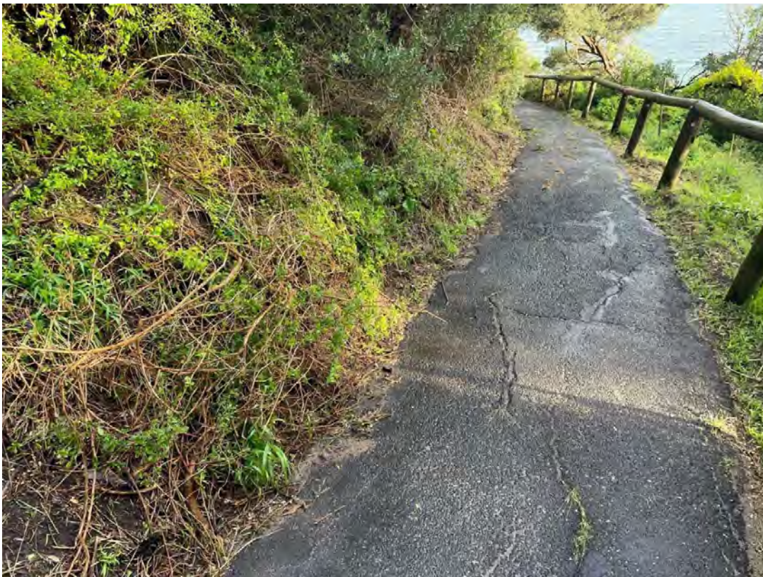
Figure 4-5 – Example of path cut into the cliff (Section 4)
