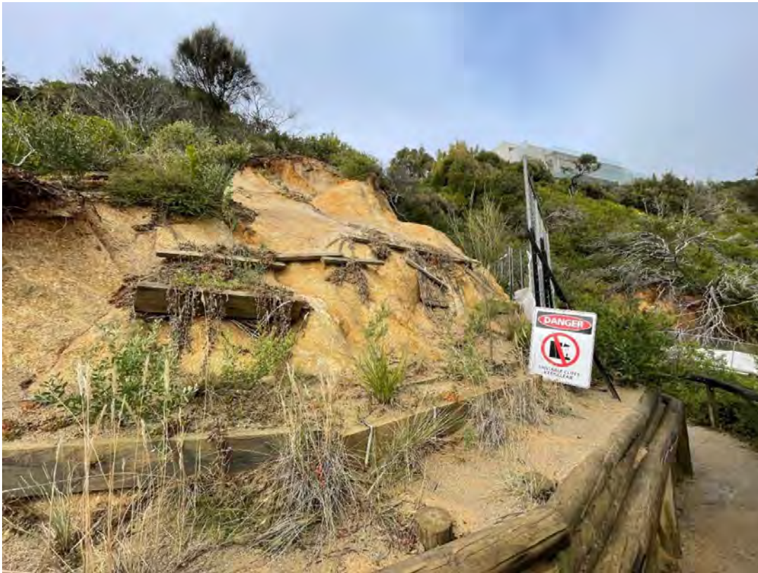
Figure 4-10 – Full and planted catch walls (Section 19)
