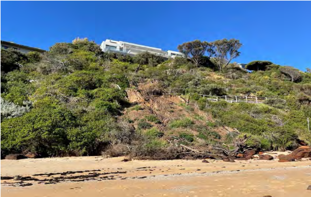
Figure 4-12 - Section 20: Recent Landslide
