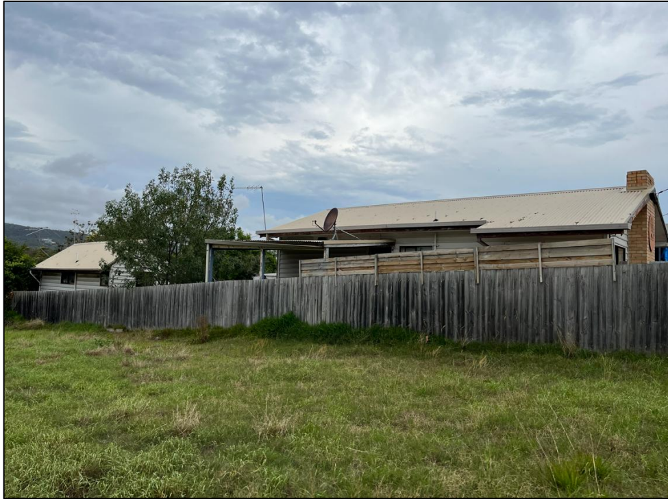
Image 4. Southern boundary of the subject site
