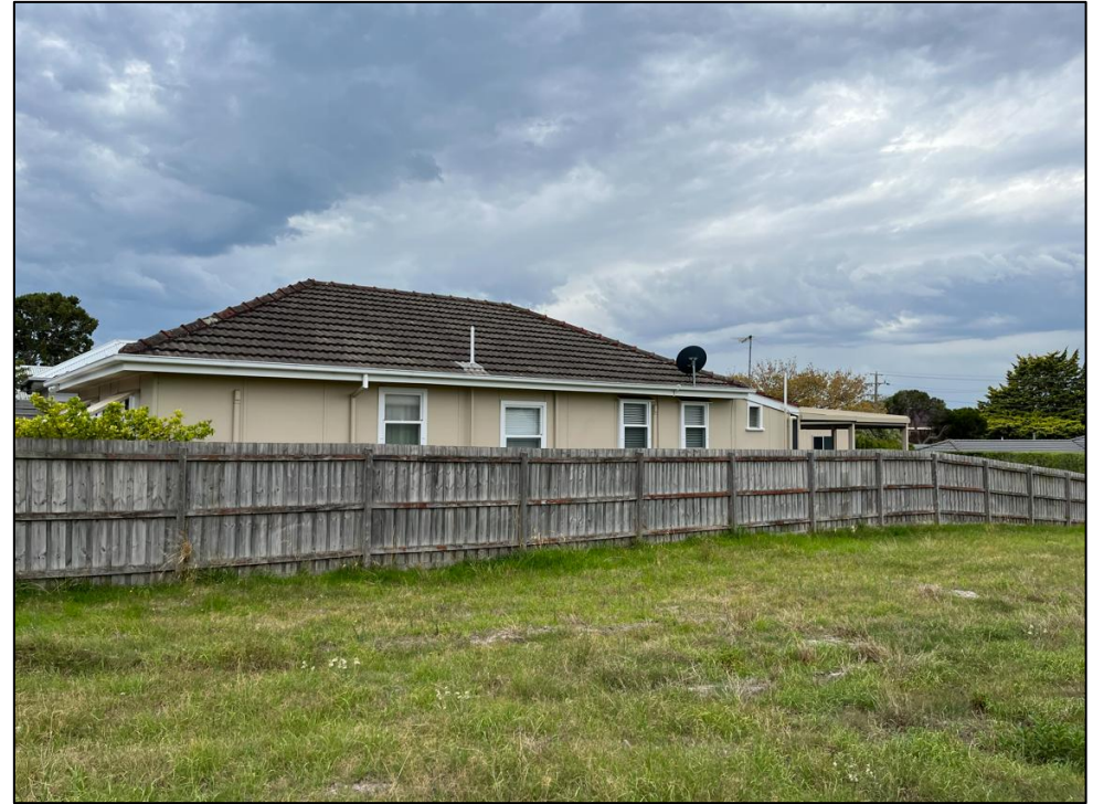
Image 5. Northern boundary of the subject site
