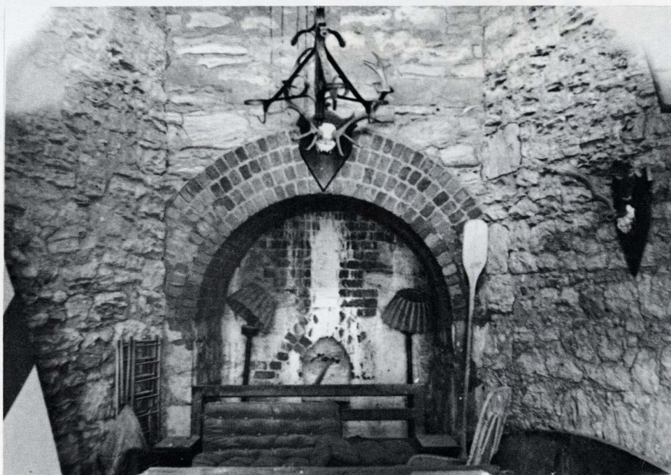
XXIX. a. & b. Breastwall and base of a lime kiln on Shelley Beach, Sorrento, Courtesy Nepean Historical Society.
