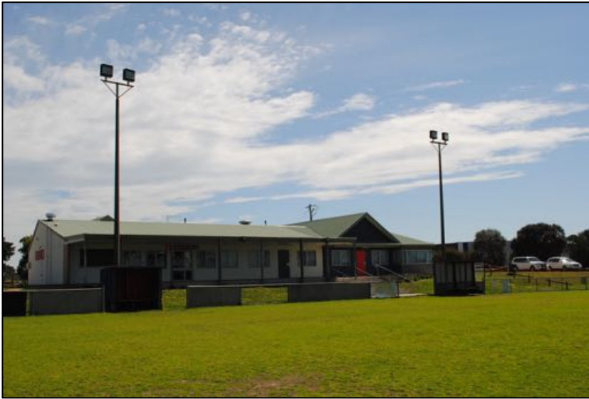
Oval 1 Floodlights and Pavilion
