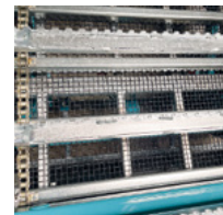
Screening sheet metal
