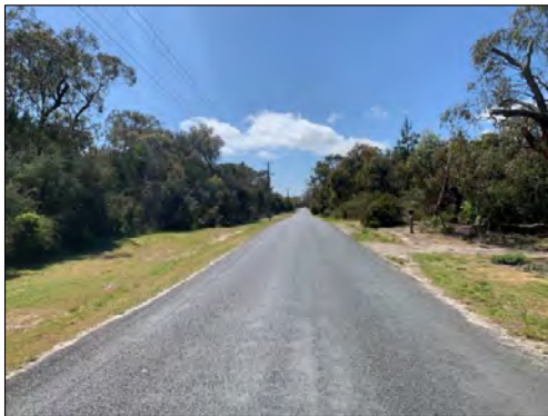
Figure 4: Lumeah Road - view east
