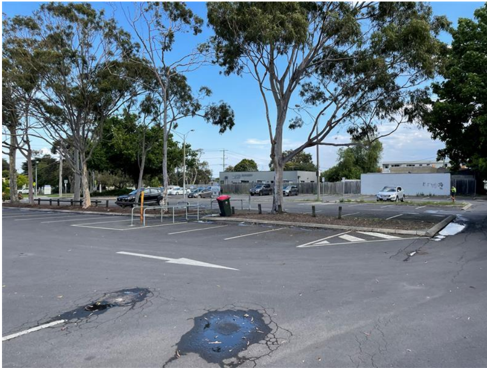
Figure 12: South-eastern facing perspective of the rear car park (156 Salmon Street).
