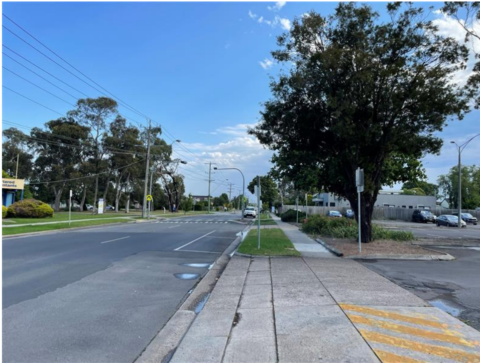
Figure 1: Southern facing perspective of Salmon Street from 156 Salmon Street, Hastings (rear car park).
