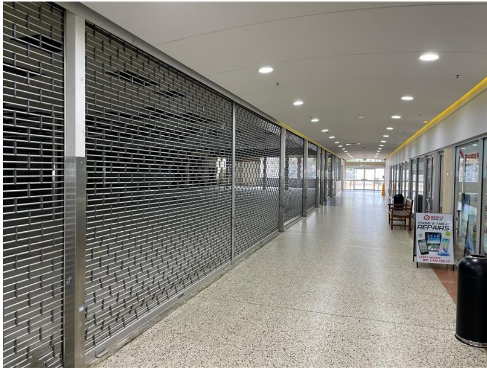
Figure 3: Southern facing internal perspective of the Coastal Village Shopping Centre with the subject premise shown (left).
