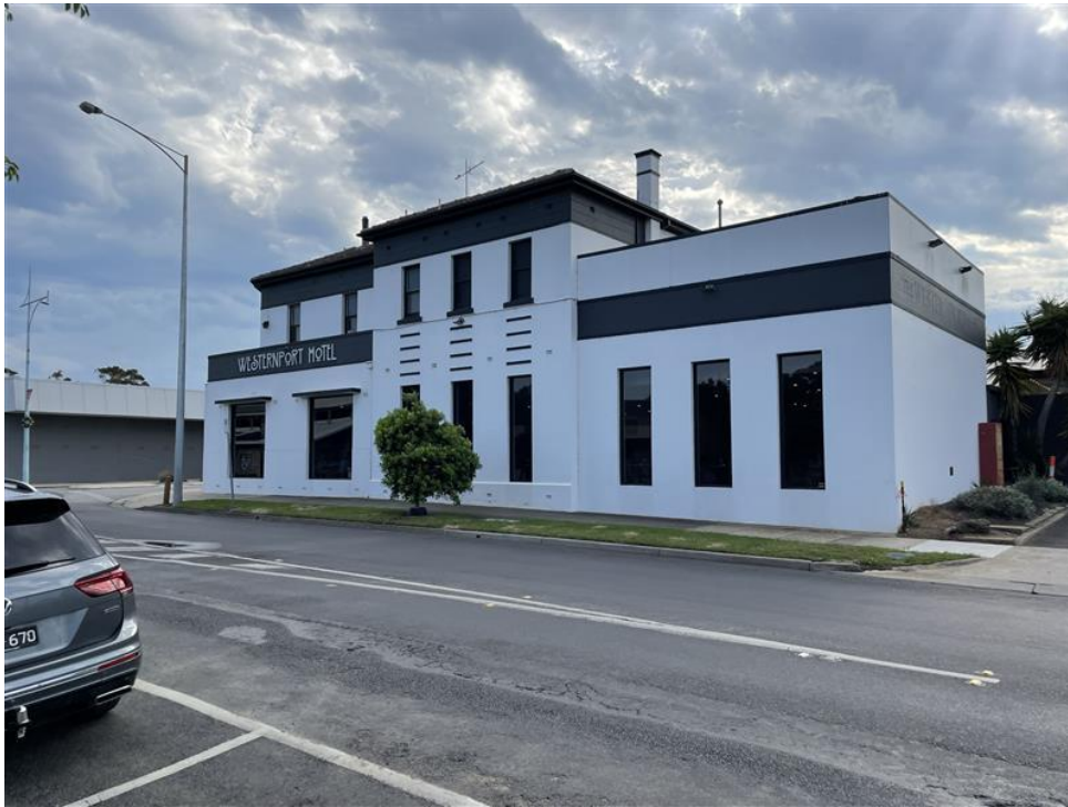
Figure 22: South-eastern facing perspective of 16 High Street (Westernport Hotel) from 4 High Street.
