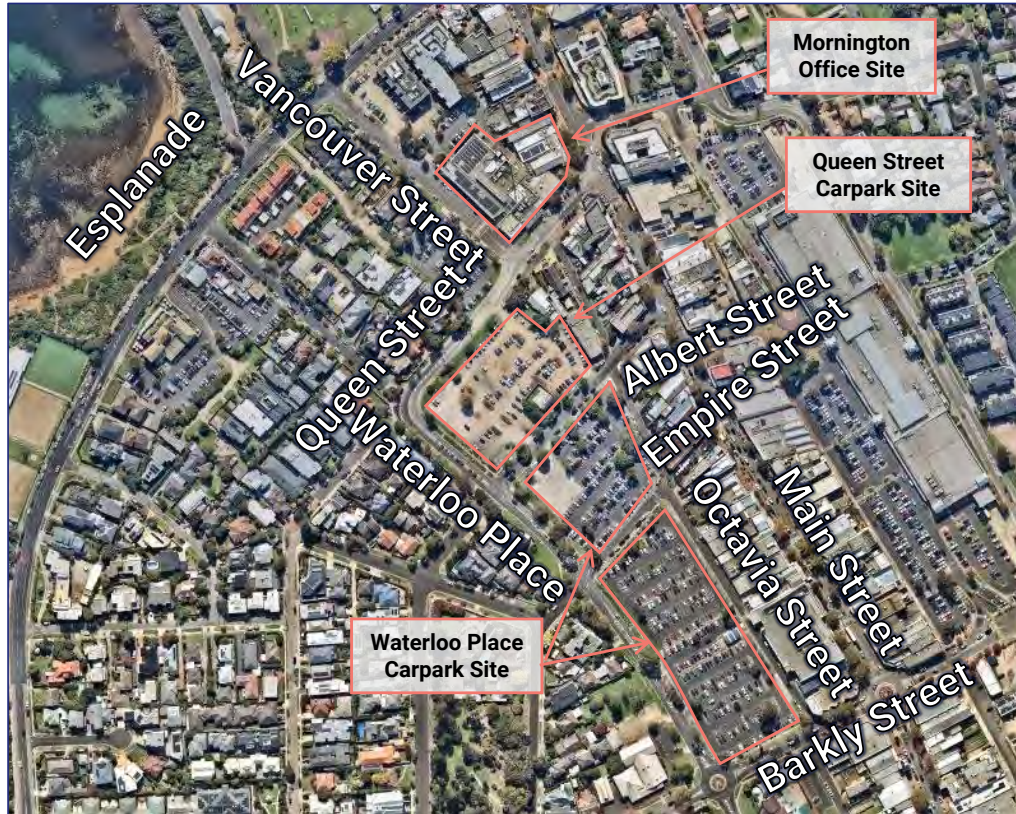
Figure 7: Aerial Photograph of Mornington Activity Centre (Source: Nearmap)
