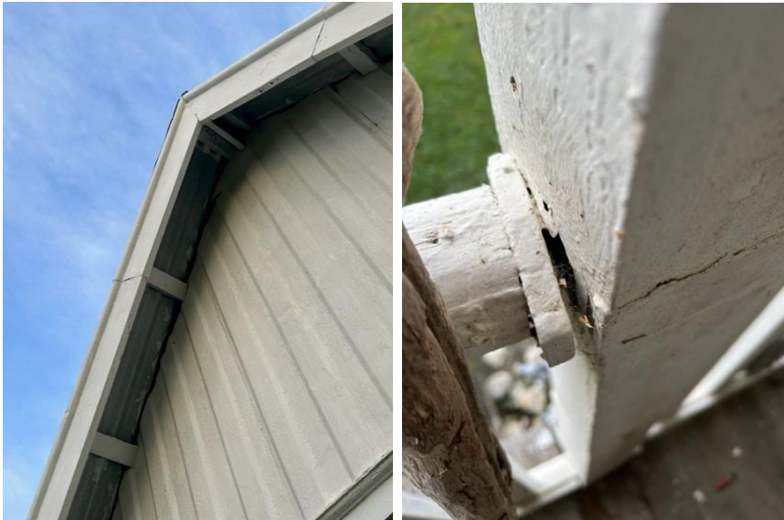
Entire front section failed, and temporary section added to replace rusted section. Balustrading totally failed.
