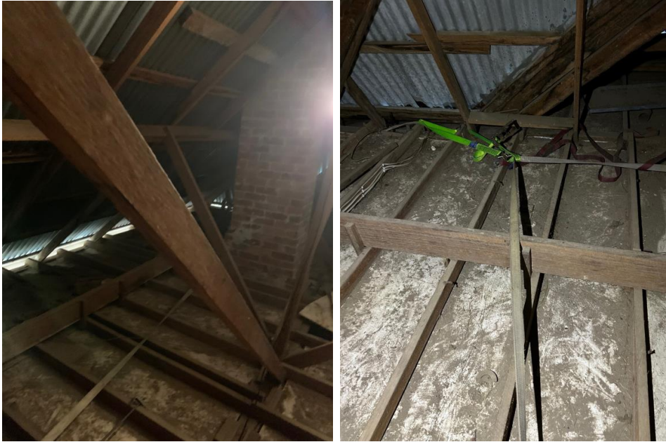
Additional bracing props to temporarily lock up the roof structure.
