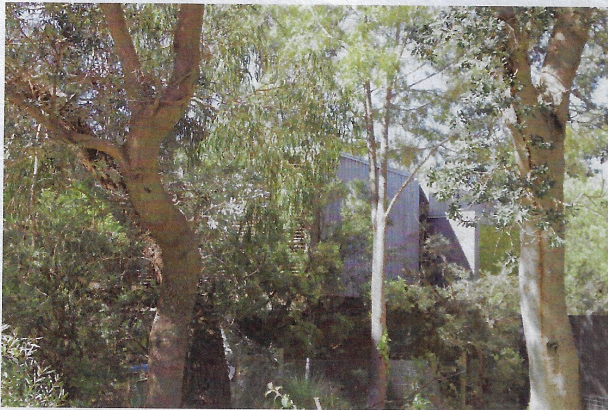
South elevation (Source: RBA, October 2022)
