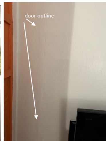
Covered door to Kitchen.
