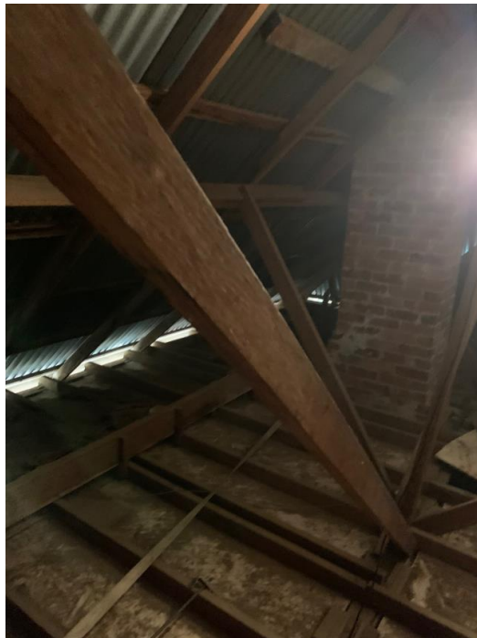
Additional bracing props to temporarily lock up the roof structure.
