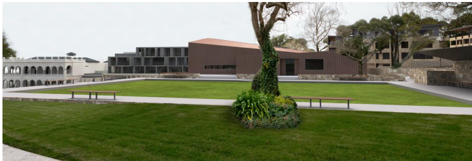
Figure 22 Place of worship (central position in background of image, with brown roof, and behind bowling green, in foreground), view from southern driveway looking north
