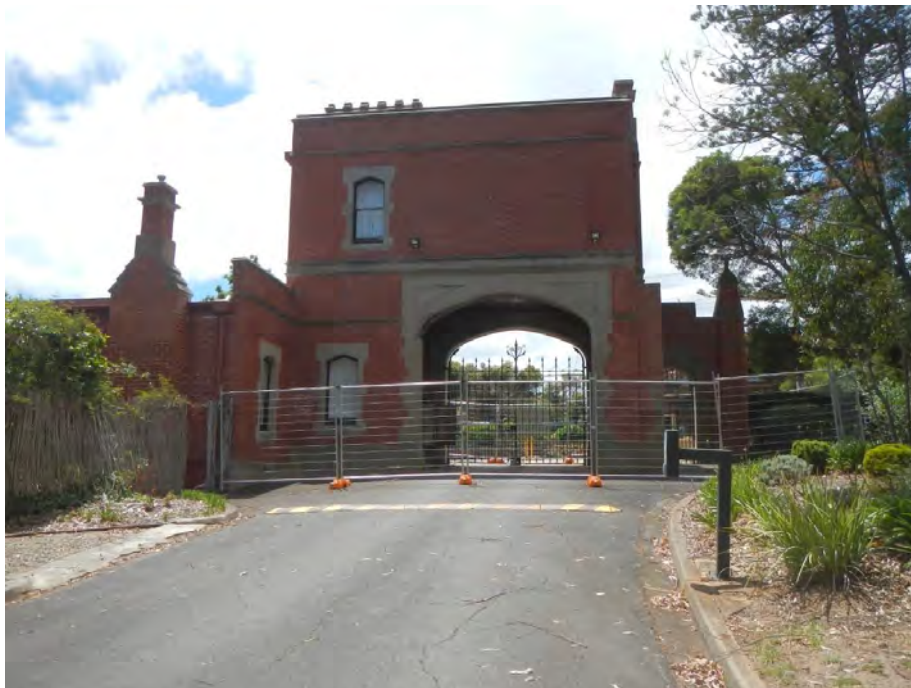
Photo 17 Gatehouse entrance from Kunyung Road, east aspect. Taken by Jodie Mitchell on 10 December 2018.
