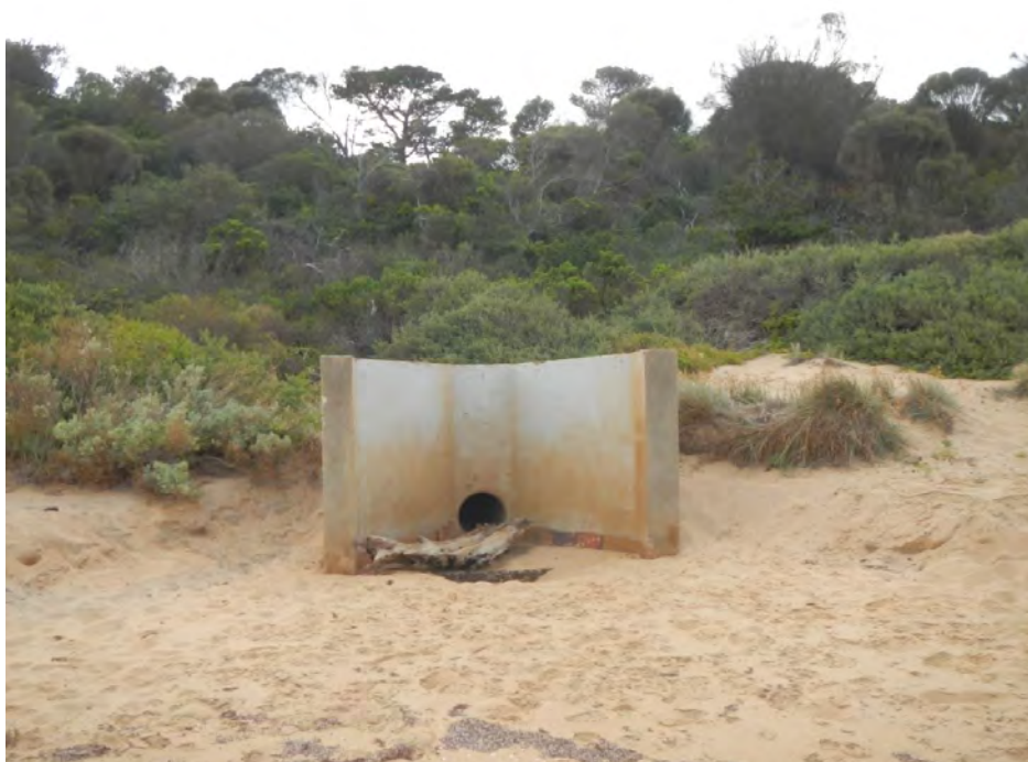
Photo 3 Concrete storm water outfall drain in beach area, east aspect. Taken by Jodie Mitchell on 10 December 2018.
