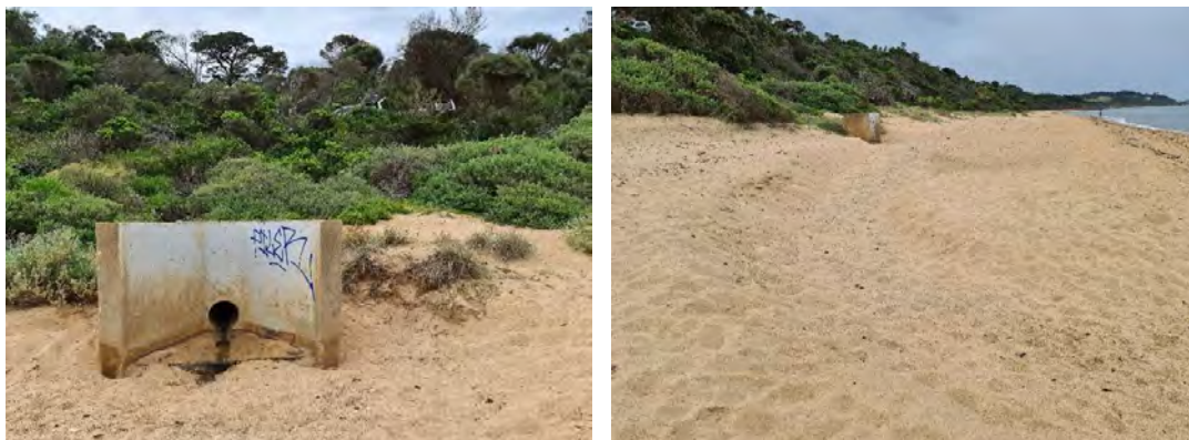
Figure 6 & 7 – Existing site discharge headwall at Moondah Beach (November 2020)
