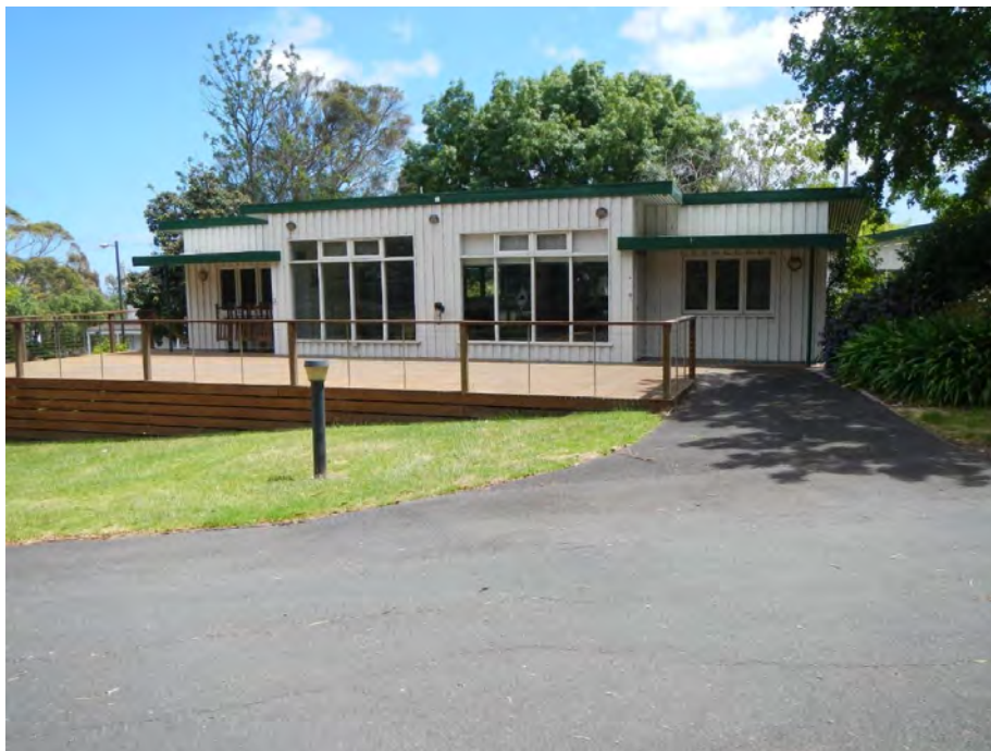
Photo 13 Demountable building north side of activity area, north aspect. Taken by Jodie Mitchell on 10 December 2018.
