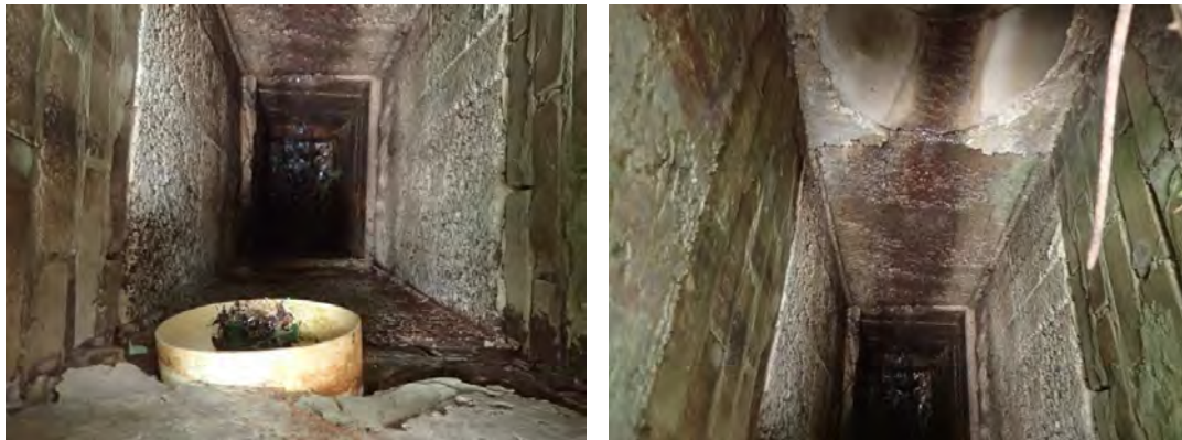
Figure 8 & 9 – Existing drainage ‘drop structure’ (November 2020)
