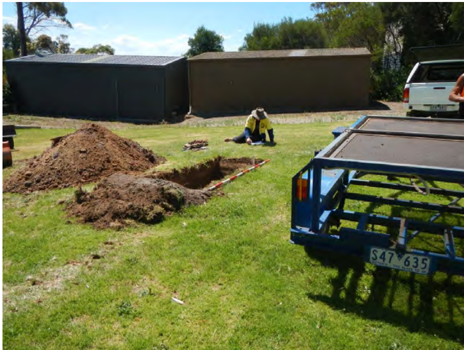
Photo 26 Location shot of MP15, north west aspect. Taken by Jason Gay, 12 December 2018
