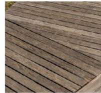
WEATHERED TIMBER BOARD WALK AND RAMP
