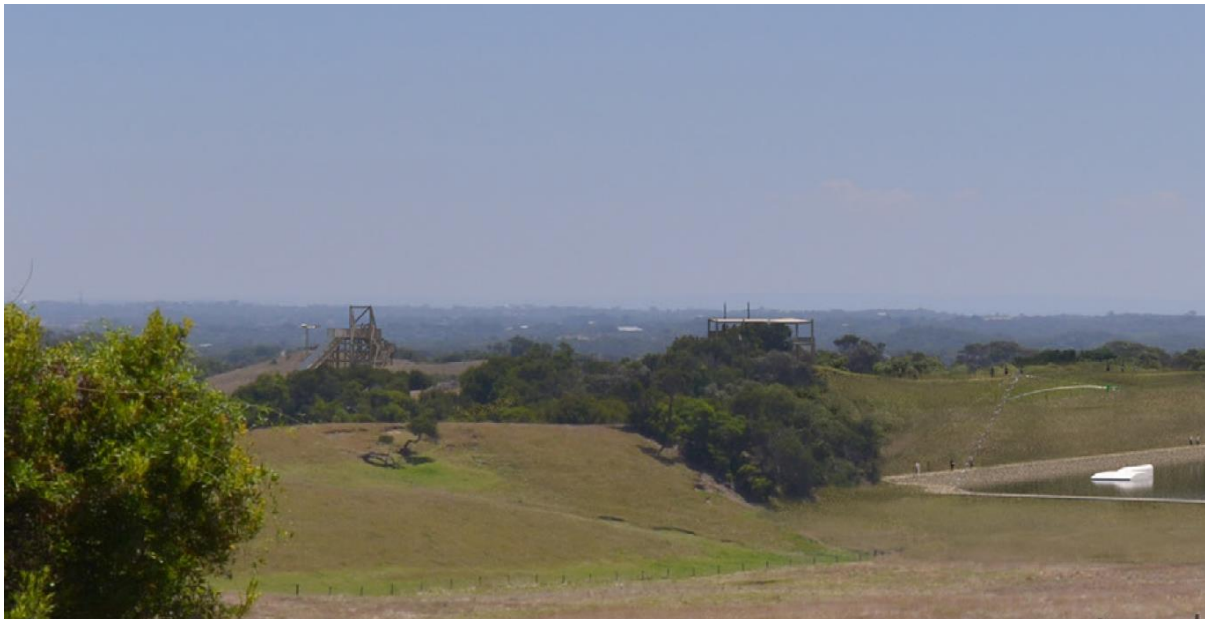
Figure 7: Zoomed-in proposed landscape as depicted in the LVIA. B12 is on the left and B11 is on the right.
