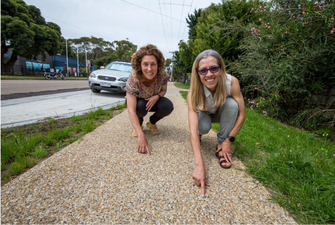
Image: Councillor Race and Councillor O Connor, pointing to a new footpath made with Replas' Polyroc
