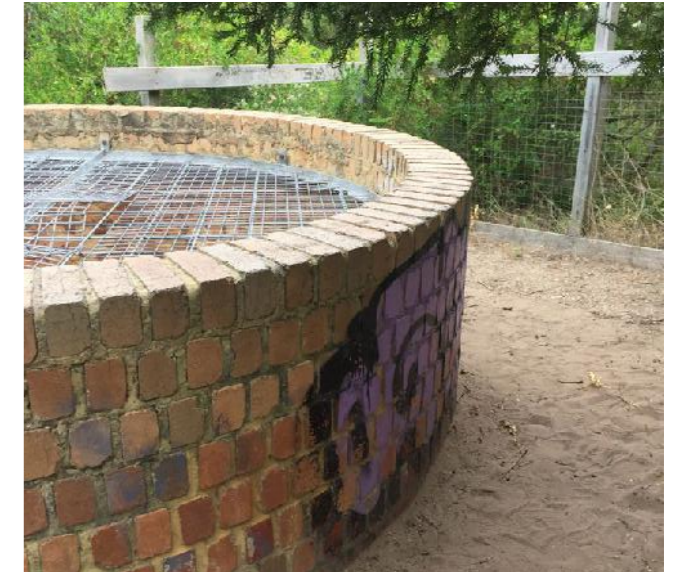
BRICK FINISH OF LIME KILN
