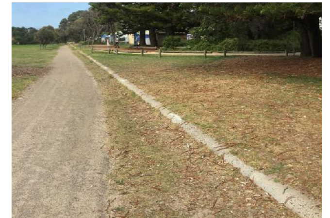
RYE HISTORIC SEA WALL
