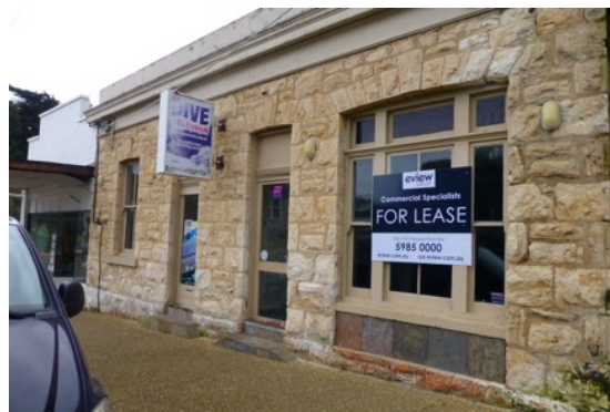
Figure 7 Limestone shopfront, Portsea
