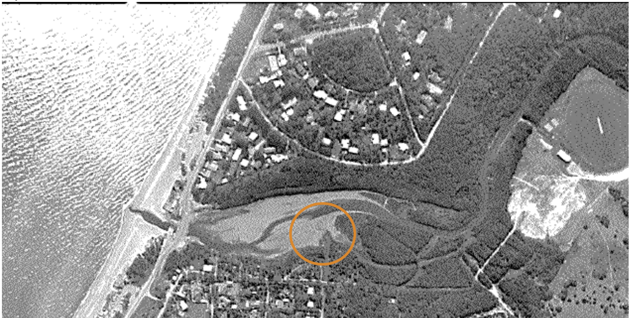
Figure 14. September 1985 historical aerial imagery (courtesy MPSC) – orange circle identifying area at the end of Henley Avenue – bayhead delta form establishing
