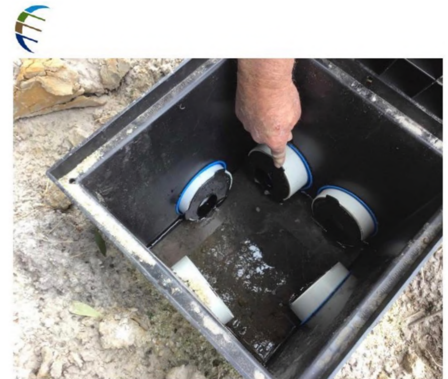
Figure 3 Adjustable Polylok weirs in place - adjust by turning tab on Rotoflow.
