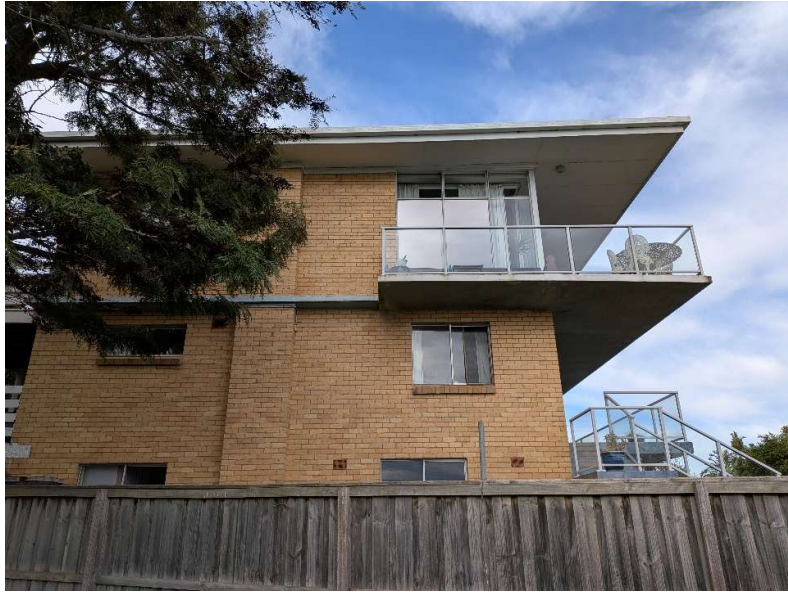
17. Adjoining dwelling, 11 Earimil Drive
