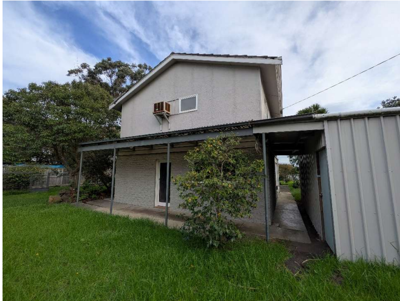
21. Existing dwelling, eastern elevation
