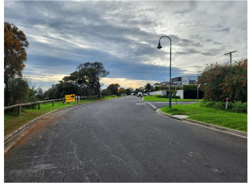
7. Facing north along Earimil Drive
