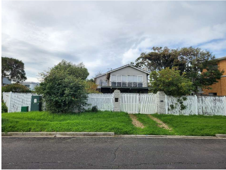
9. Western façade, Earimil Drive
