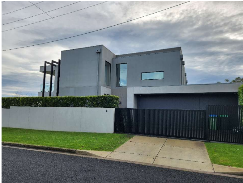
6. Opposite the Site to the north, 13 Earimil Drive
