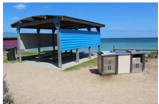
Existing BBQ facility and picnic shelter
