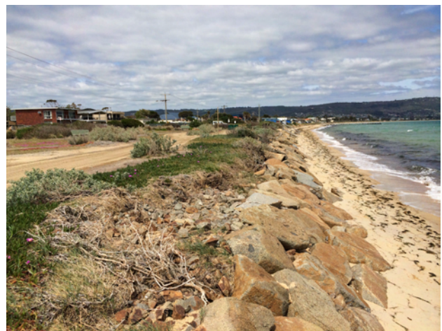
Rock stabilized slope between beach and reserve
