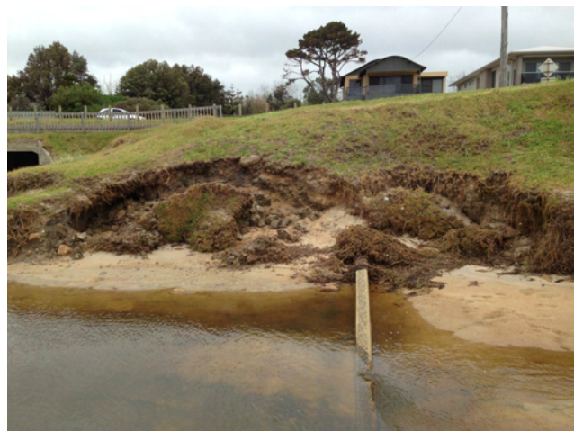
Erosion at mouth of Dunn's Creek
