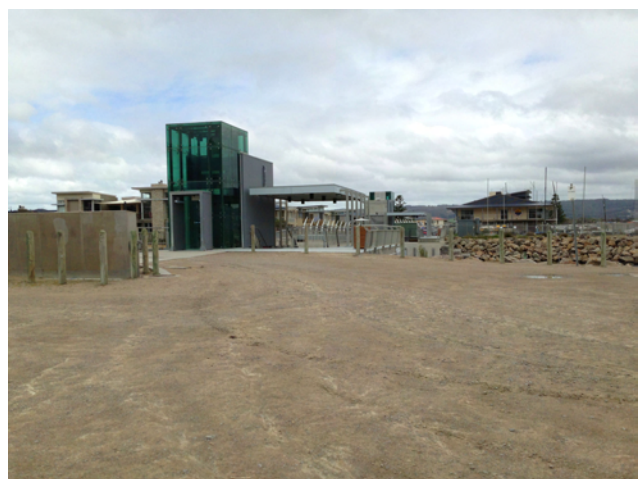
View of Martha Cove Lift/stairwell and carpark area
