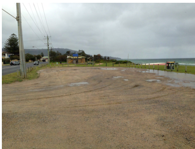
Large informal Gravel carpark near Prescott Avenue
