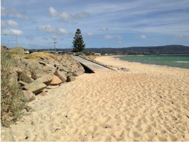
Disabled Beach Access ramp at Community centre
