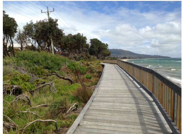
Existing Boardwalk through Banksia woodland area.
