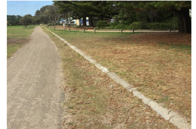
RYE HISTORIC SEA WALL
