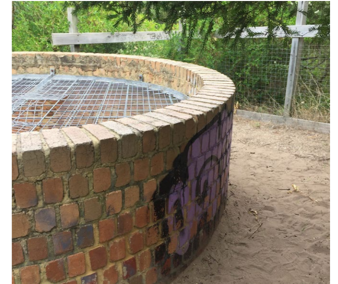
BRICK FINISH OF LIME KILN
