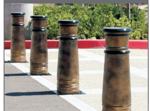
The use of 'flush' pavements and bollards to delineate traffic and pedestrian areas promotes continuous accessible paths of travel.
