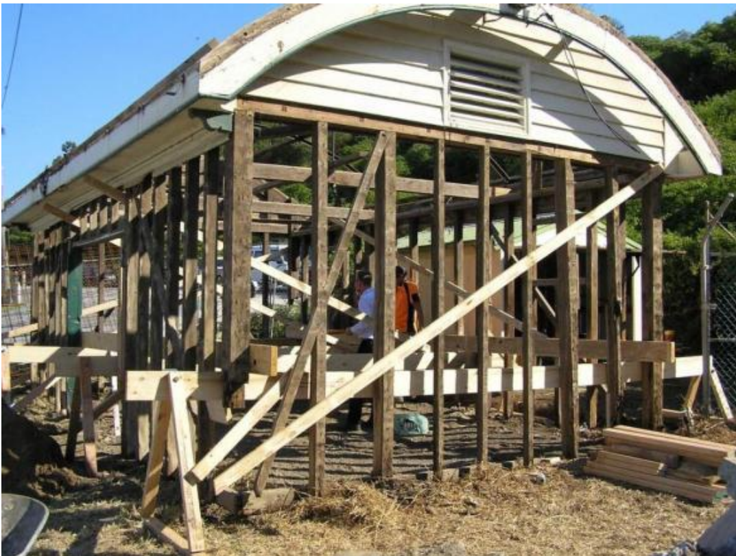
Figure 52: Cargo Shed during restoration (Photo Lorraine Huddle 2010)
