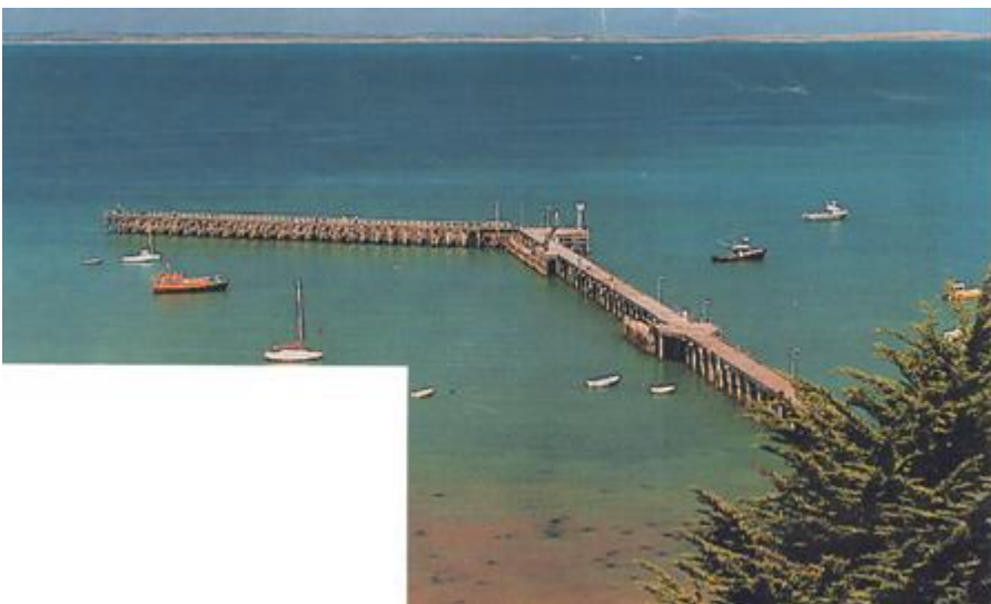
Figure 35: Flinders Pier prior to demolition of breakwater (URS 2008)
