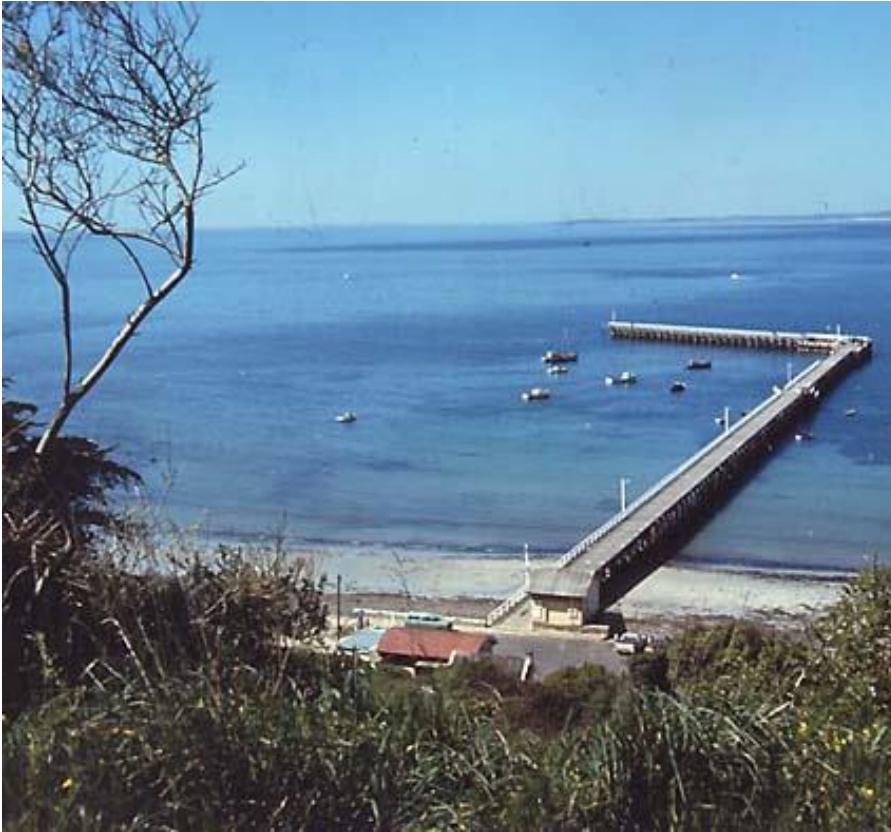
Figure 34: Flinders Pier showing the dogleg section and original location of the smaller shed 1971 (National Library of Australia, NAAA1500, K26763)
