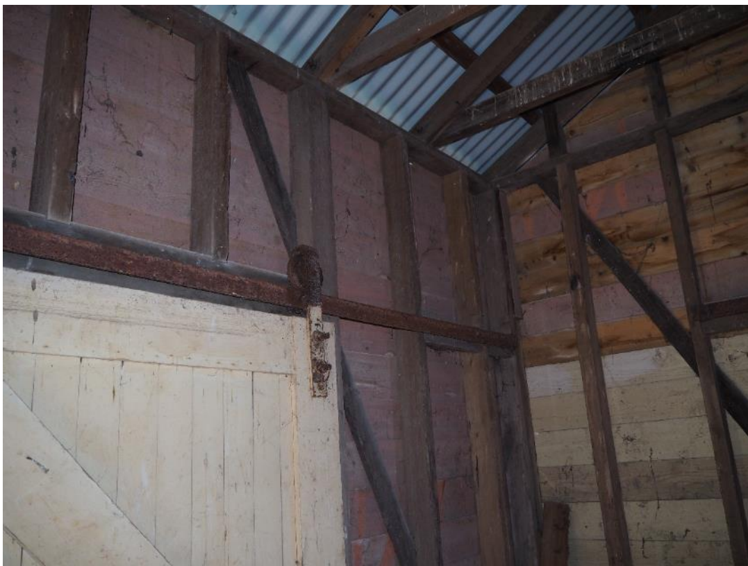
Figure 83: Interior of shed showing various stages of weatherboard replacement.
