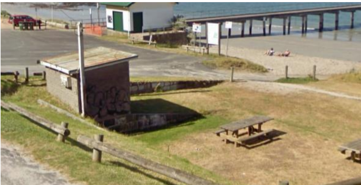
Figure 59: Slipway Winch shed from above retaining wall (G. Vines 2013)
