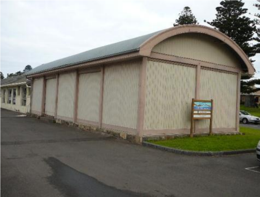
Figure 73: Port Fairy wharf shed, note panelled construction form with expressed posts 106
