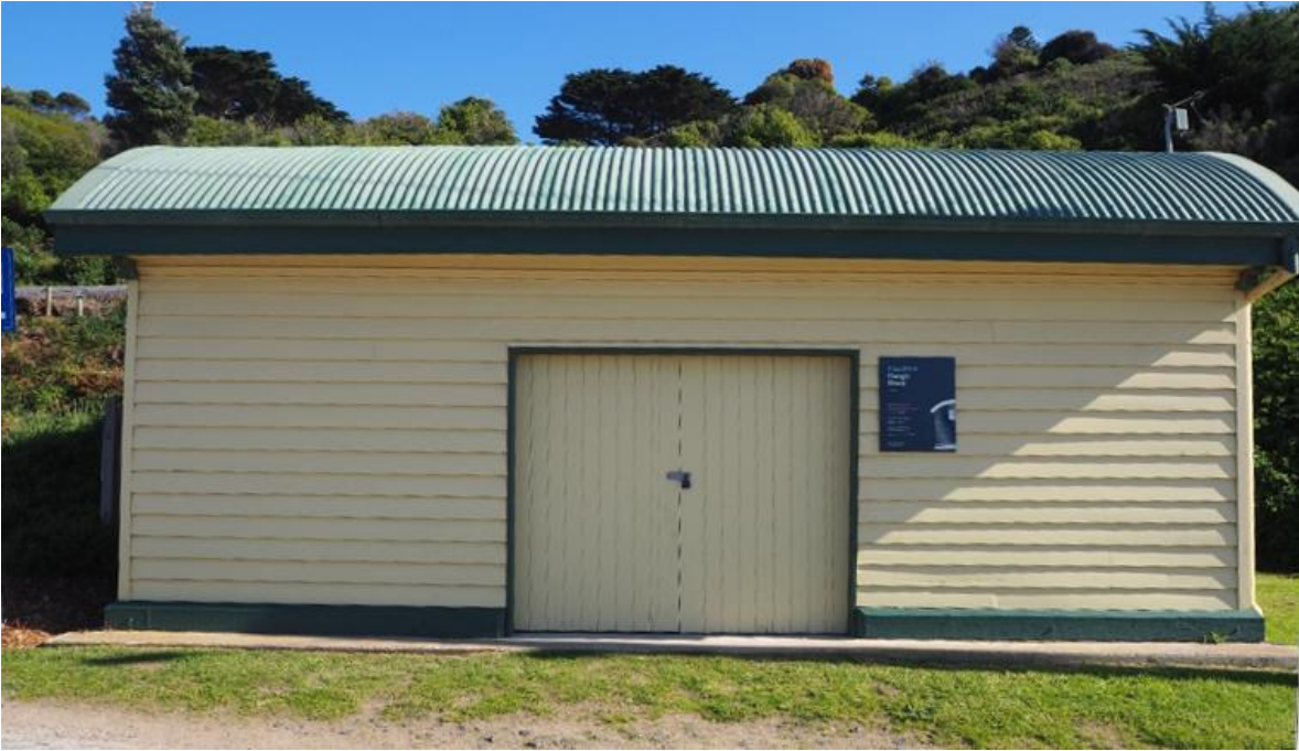
Figure 53: 1871 Cargo Shed following restoration (G. Vines 2023)
