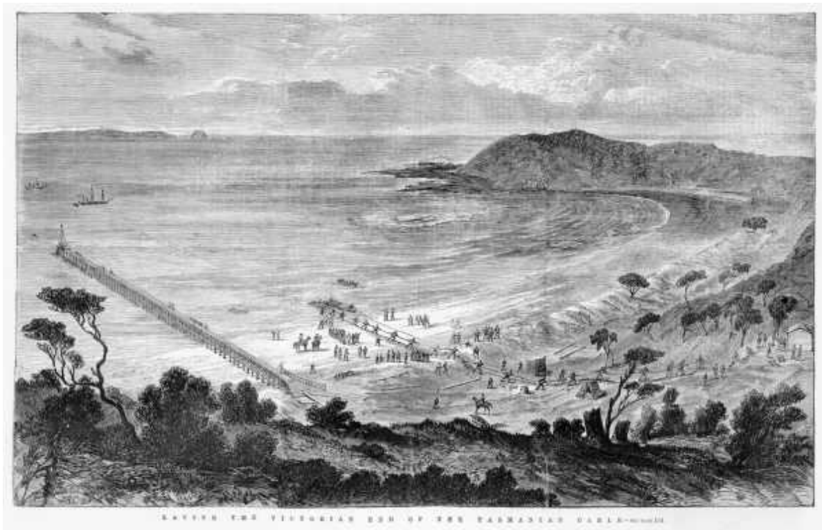
Figure 17: "Laying the Flinders end of the Tasmanian Cable" (SLV mp001494). 43
