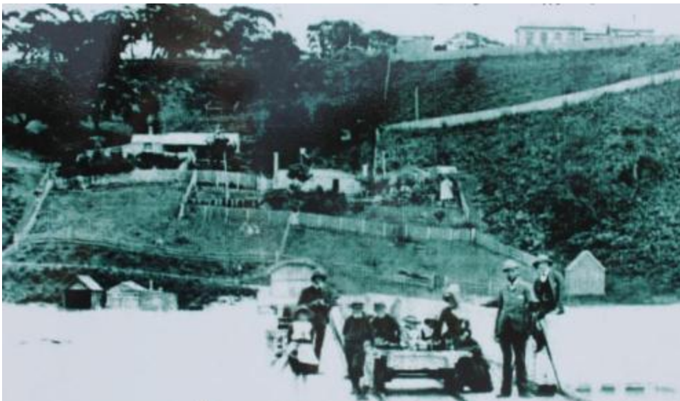
Figure 29: Trolley on the pier tramway with cable station behind (Photo Flinders Historical Society from interpretive sign)
