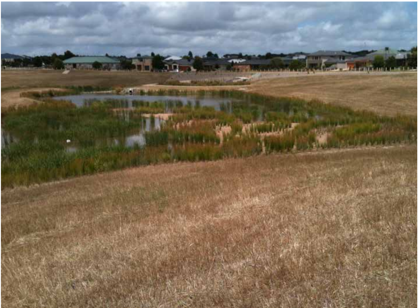
Large scale Tanti wetlands - 'Flagship' partnership project between Melbourne Water and Mornington Peninsula Shire
