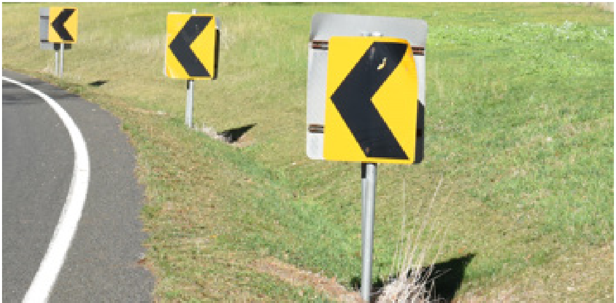
Figure 3-2 Curve Alignment Marker (CAM) Signs
