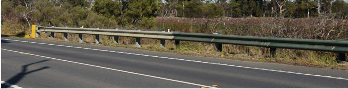
Figure 6-5 Road safety barrier along Tyabb-Tooradin Road
