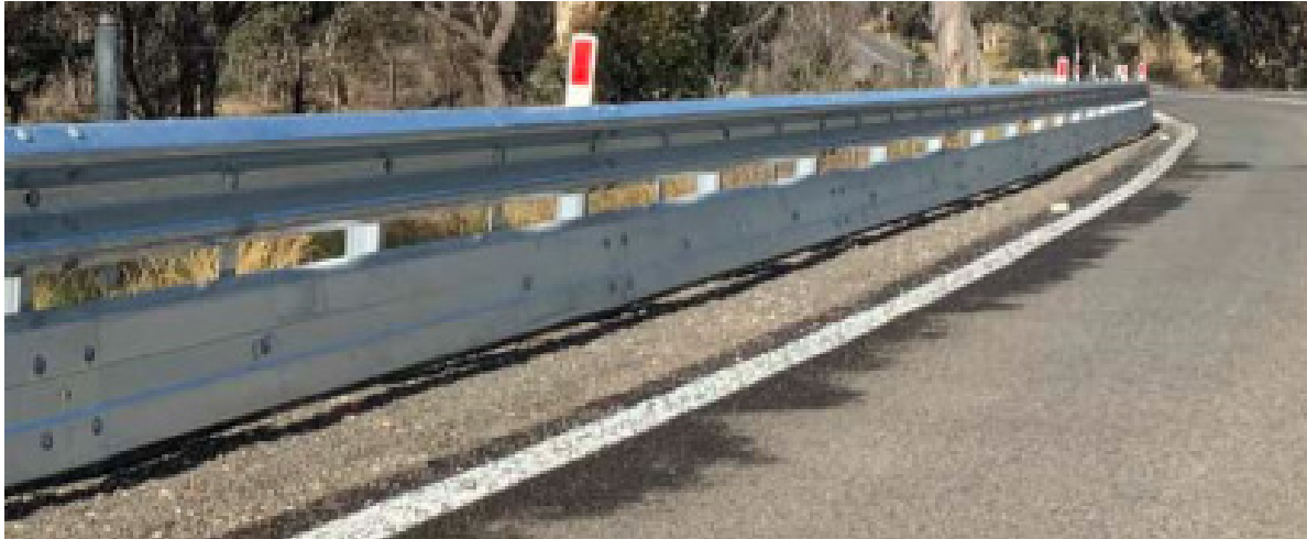
Figure 3-4 Road Barrier with Underrun Protection
