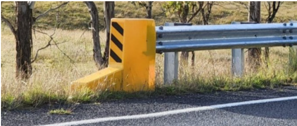
Figure 3-5 End Terminal on Road Barrier
