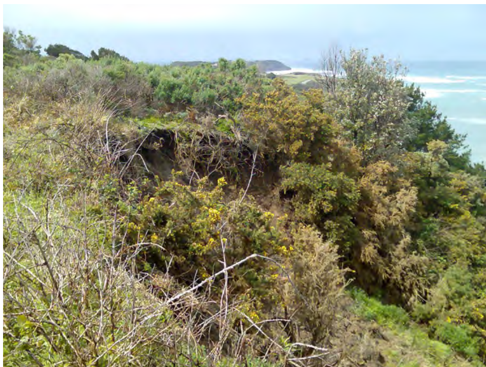
Plate 12.2: Scarp with Active Erosion and Movement
