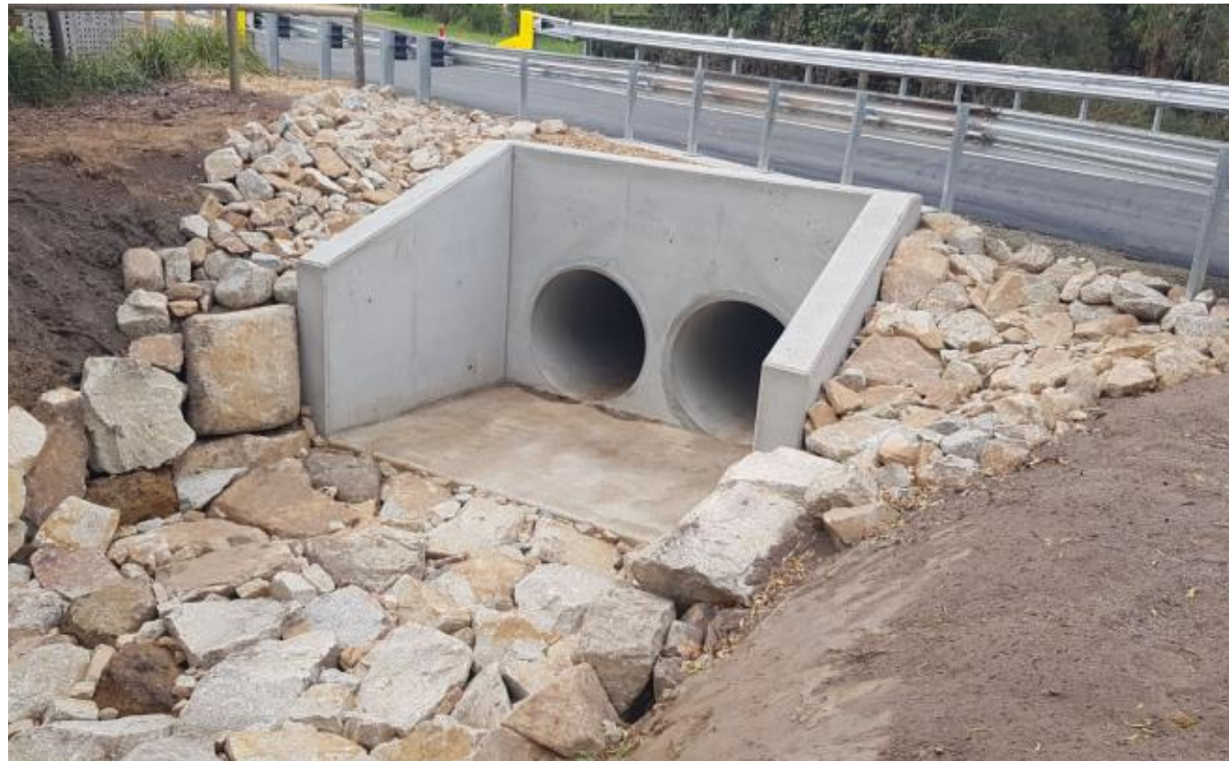
Mount Martha Briars Culvert Bridge
