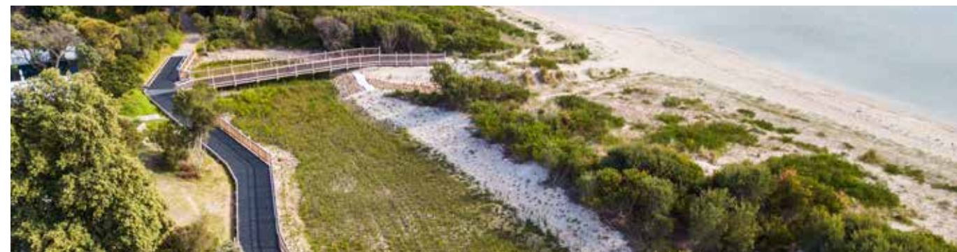
Image: Rye Coastal Wetland Biofiltration
