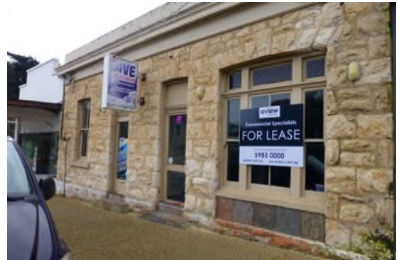
Figure 7 Limestone shopfront, Portsea
