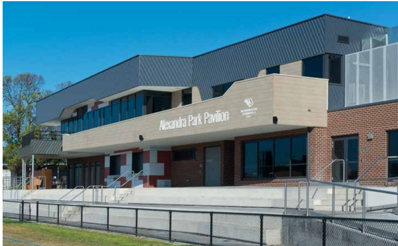
Mornington: Alexandra Park Pavilion
