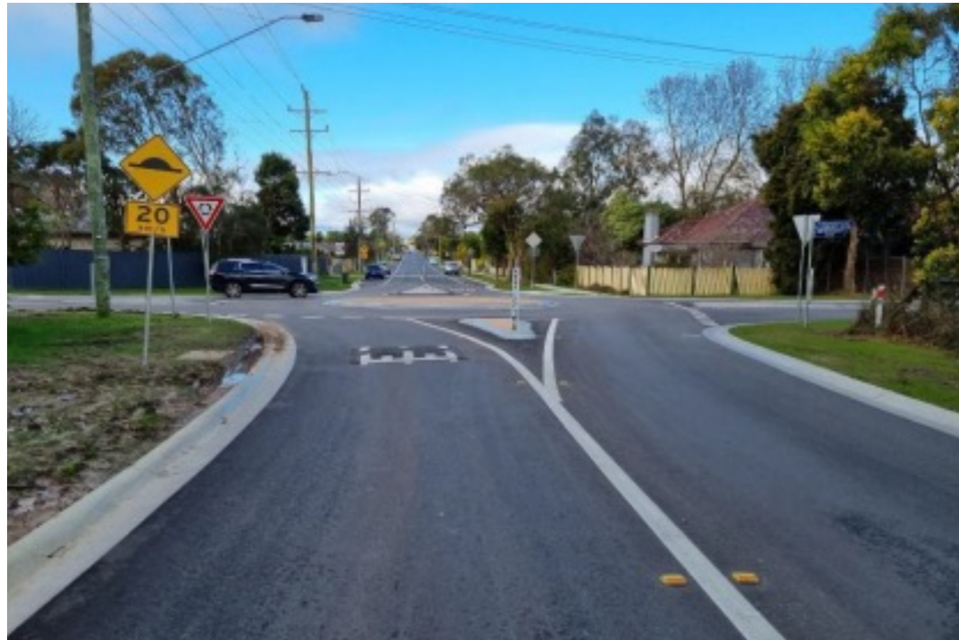
Bittern: Blackspot Program Myers/Henderson Road Roundabout Total project value $600,000
