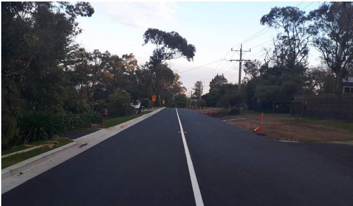
Image: Two Bays Road, Mount Eliza – Road Widening
