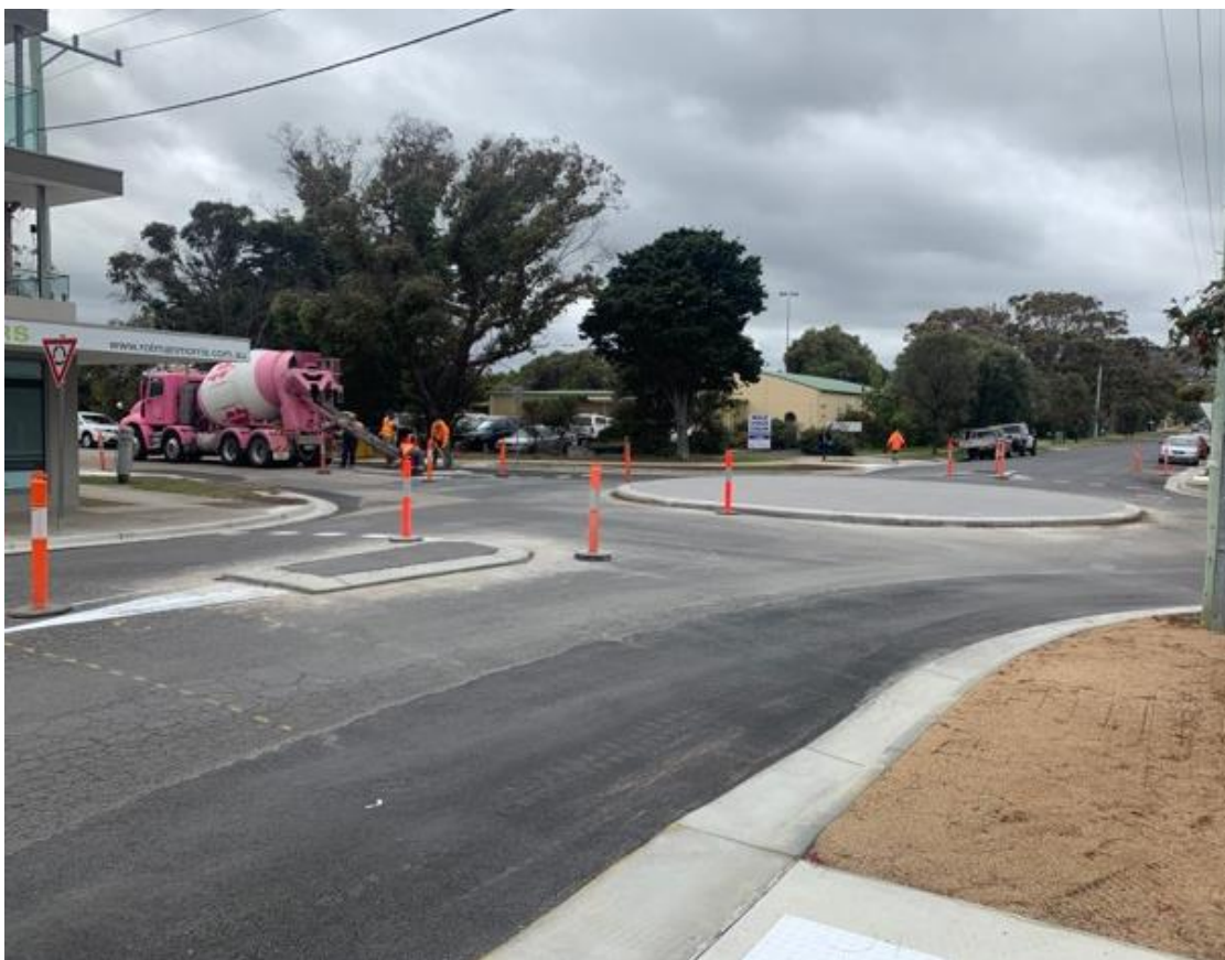
Image: Roundabout under construction at Pier Street, Dromana.
