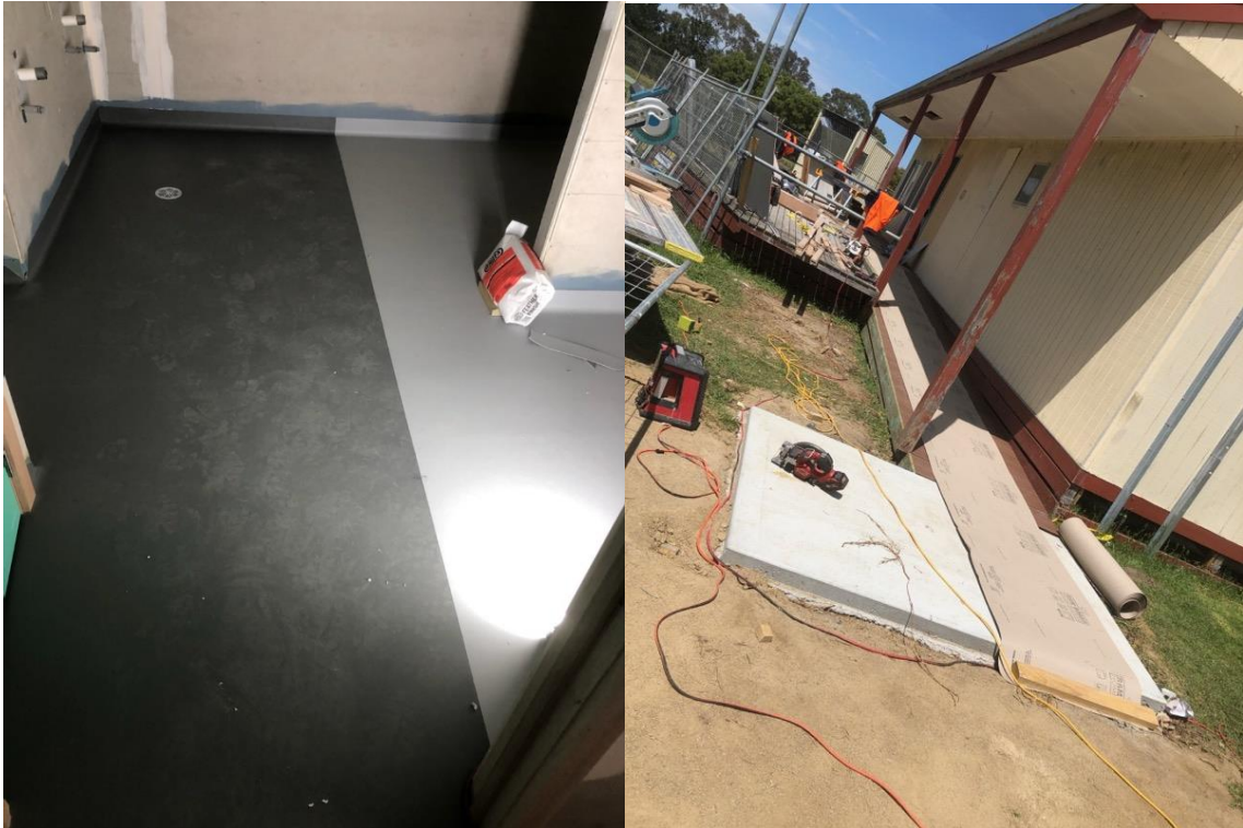
Image: internal vinyl floor coverings and external ramp completed
