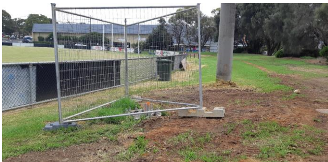
Image: Alexandra Park, Mornington – Completed light pole footing and cable trenching
