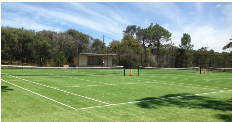
Image: Watson Road Tennis Courts close to completion
