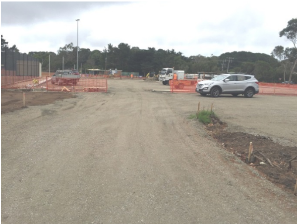
Image: current progress of works- Balnarring Recreation Reserve
