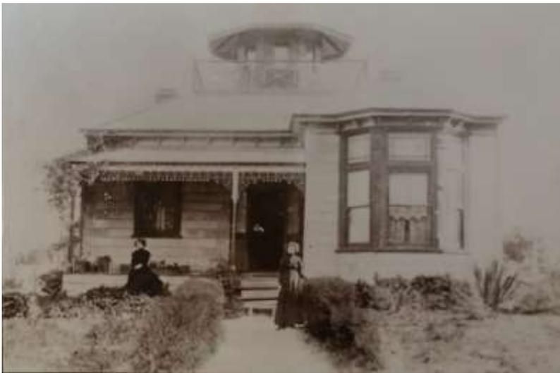
Photo: Early photo c1900 of Tower House showing the roof-top balustrade and octagonal lookout tower. Photo provided by Somerville, Tyabb & District Heritage Society.
