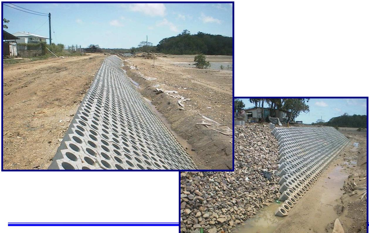
**Figure 5.2: Hexagonal block concrete seawall**
