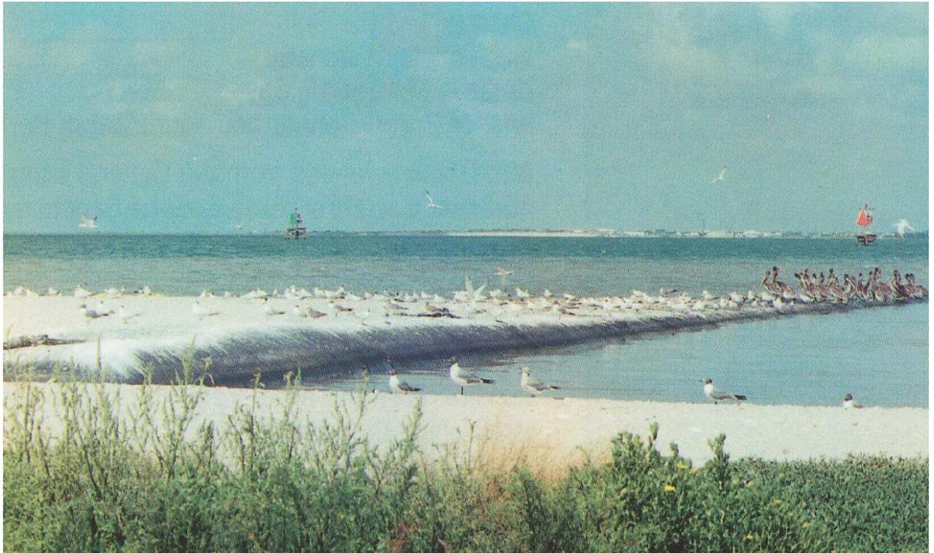
**Figure 5.3: Example of Geotextile Groyne**
