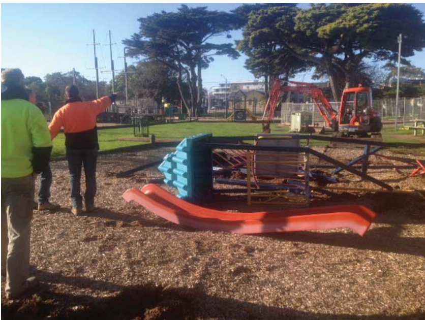
Image: Demolition of old equipment
