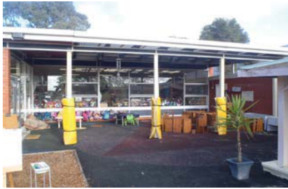
Before installation of all-weather blinds
