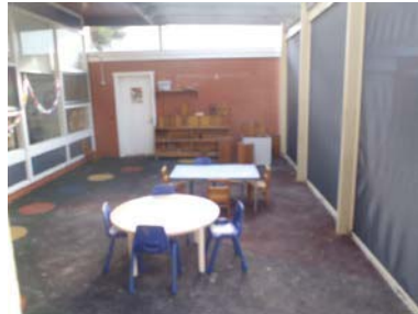
After installation of all-weather blinds
