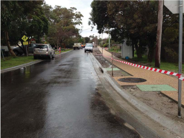
Image: Newly laid asphalt and exposed concrete footpath
