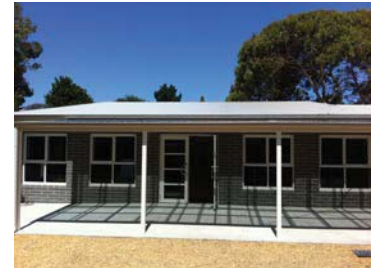
Completed veranda at Sorrento Kindergarten
