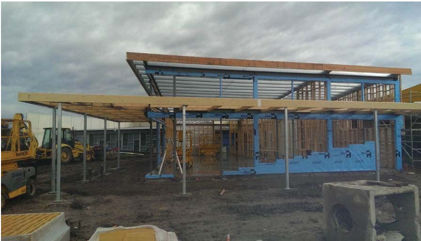
Image: Bentons Square Preschool building frame
