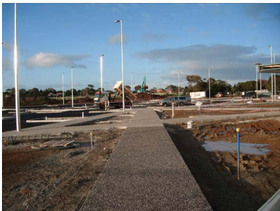
Image car park construction
