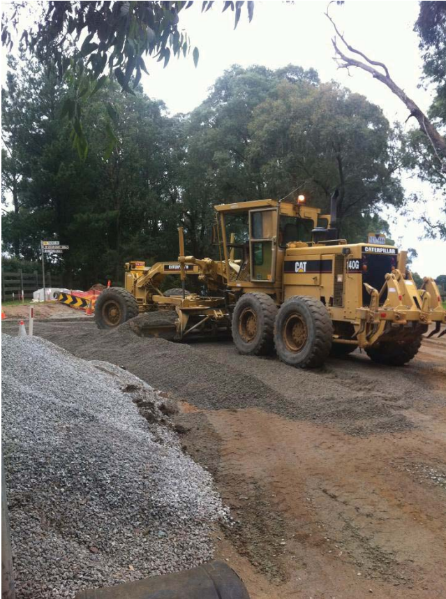
Image: Grader spreading rock at Tucks Road Intersection
