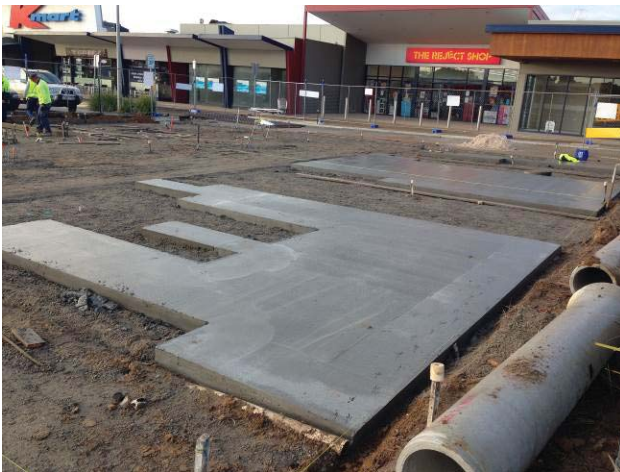
Image: Newly poured foundations for the new Streetscape Works within Alfred Street
