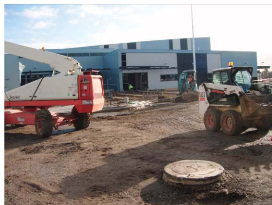
Image front entry works
