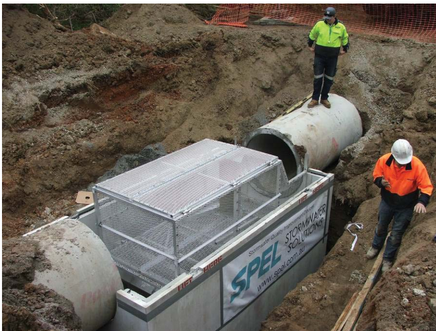
Image: New Gross Pollution Trap being installed.
