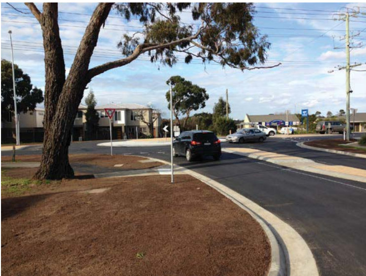
Image: newly constructed roundabout
