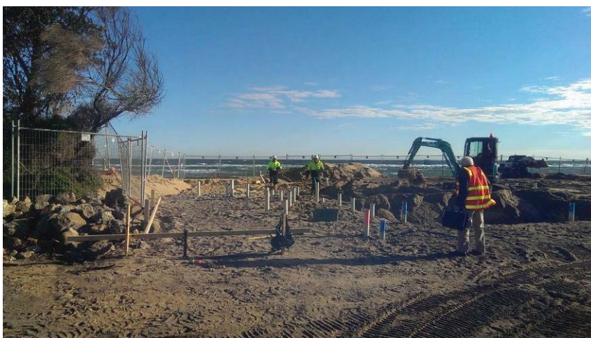
Image: Mount Martha Life Saving Club building foundation works
